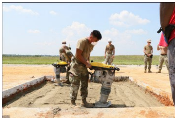
5 - Backfill
