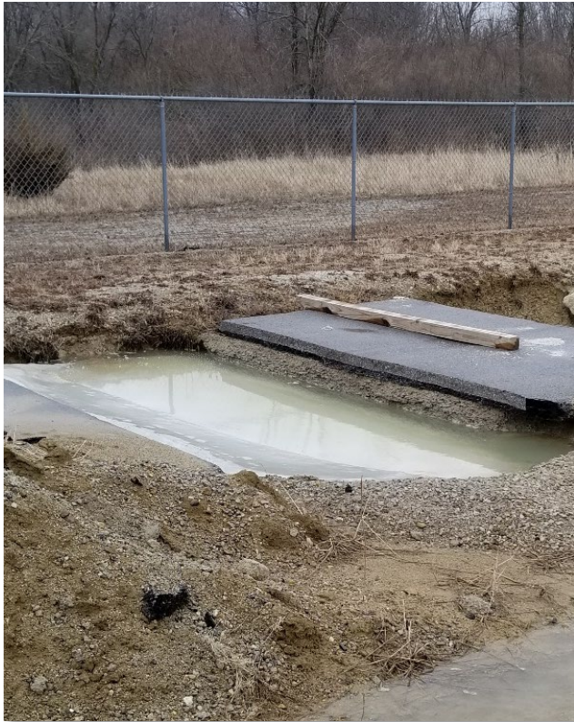
C2S3 Ice Inside Trench
