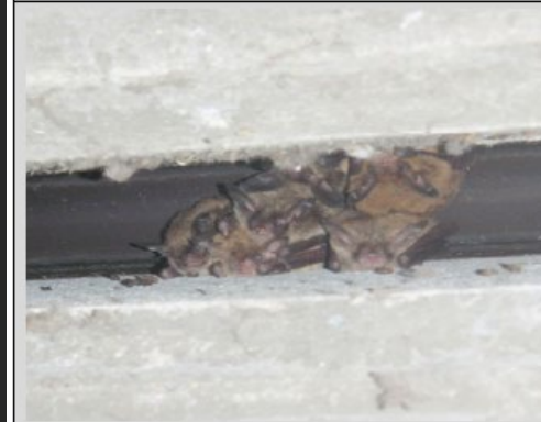
Condition State 4 Bats roosting on the underside of a deck joint
