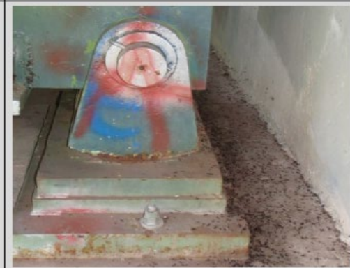
Condition State 4 Bats droppings on an abutment bearing seat
