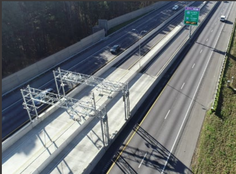
I-75/575 Northwest Corridor, Atlanta
