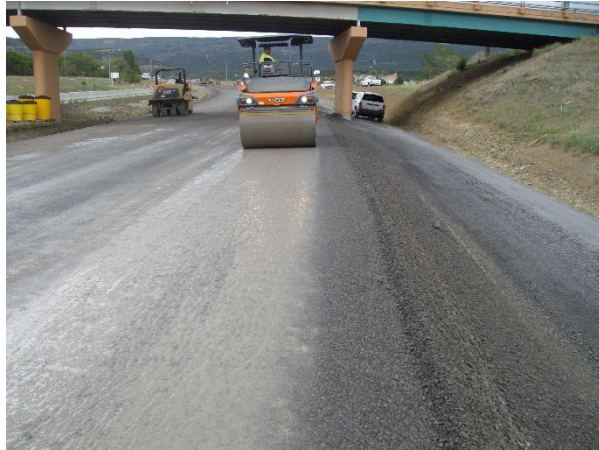
Excess Fines Expelled as Slush from Layer
