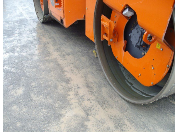
Excess Fines Expelled as Slush from Layer
