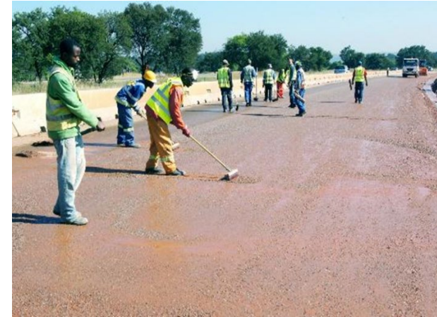
Brooming and Spreading Initial Slush/Fines to Deficient Areas
