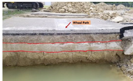
C3S2W – QB2 + Cement Subbase + CA06_R
