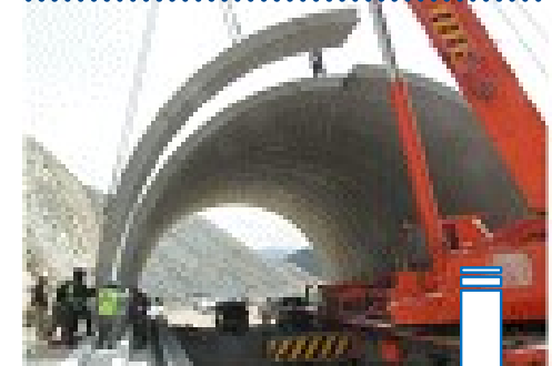
4. Arch Erection
