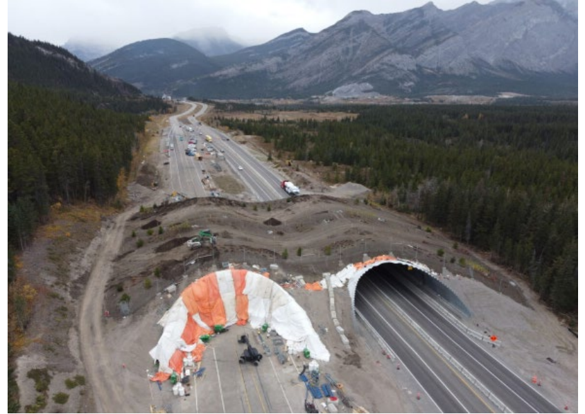
Live traffic proceeding throughout bridge construction
