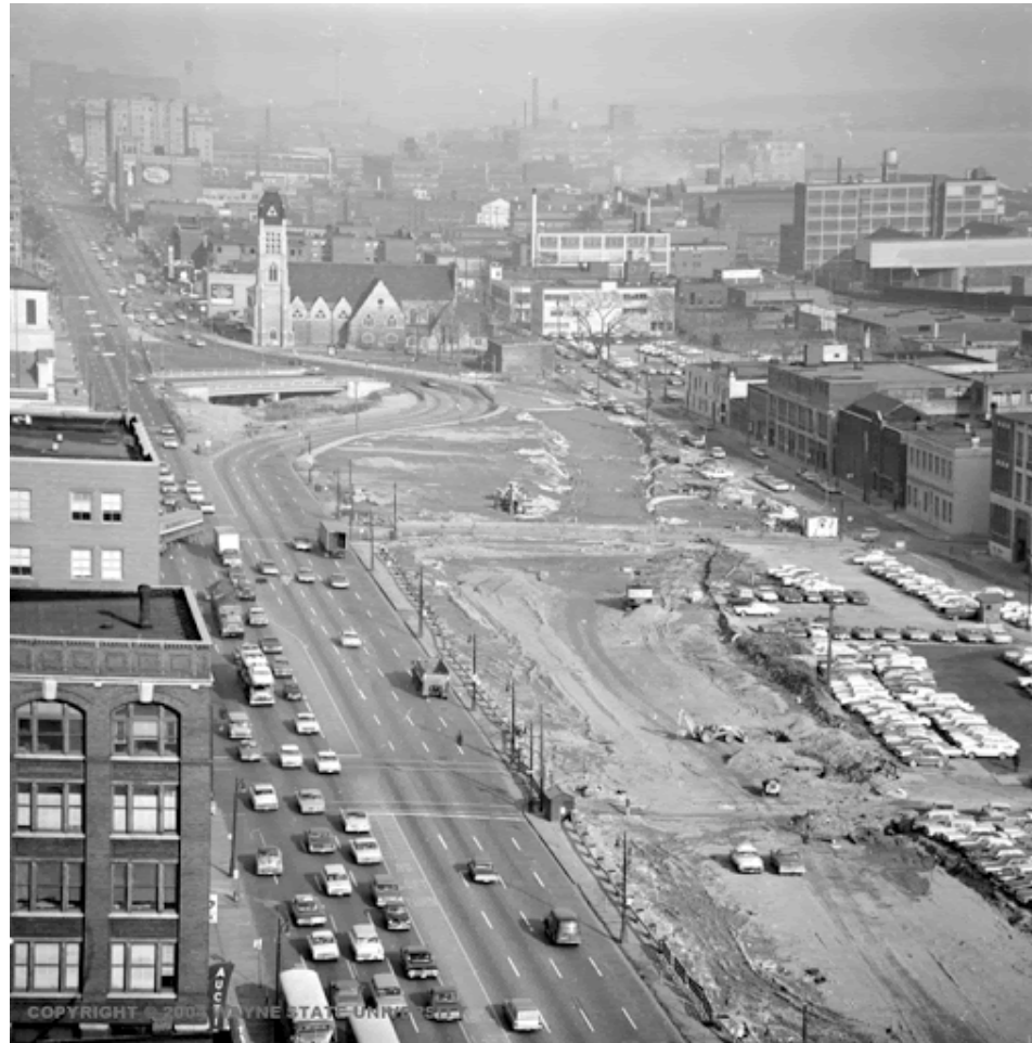
Chrysler Freeway construction in Detroit, MI
