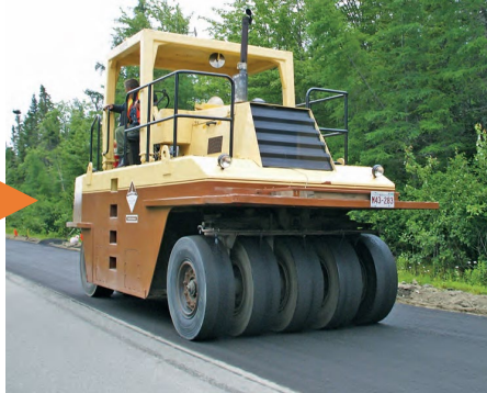
Compaction to target density
