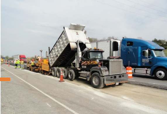
CCPR mix is loaded into asphalt paver hopper
