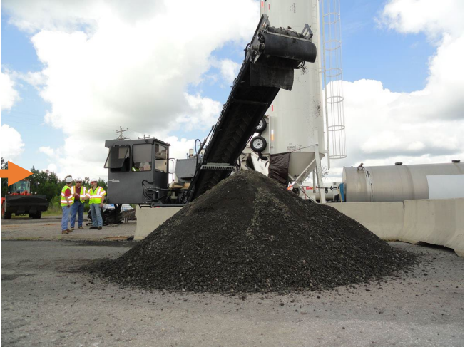
CCPR mixture discharged onto ground or into dump truck
