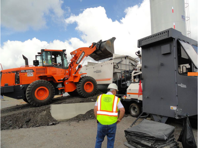
RAP loaded into CCPR plant hopper
