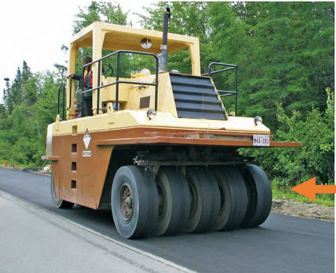
Compaction to target density
