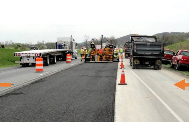
CCPR mix is paved and rolled to specification
