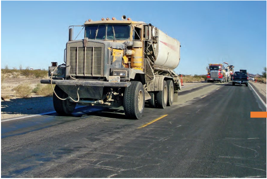
Dry additive application on pavement ahead of CIR train (if needed)
