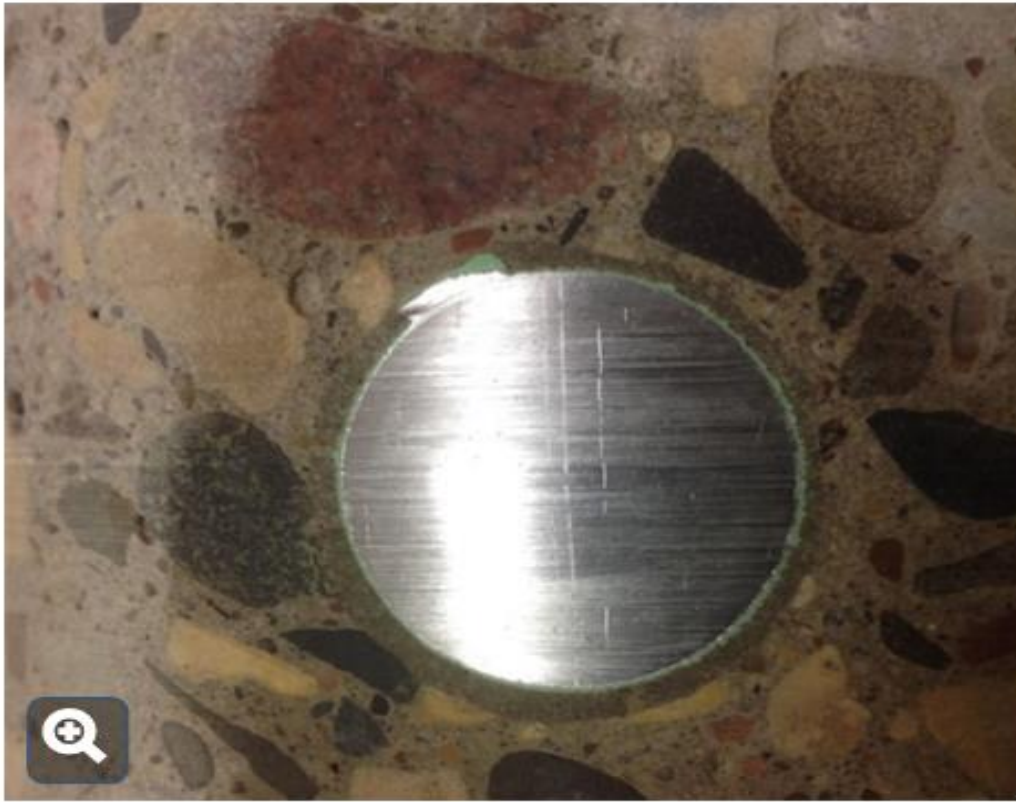
Acceptable – Grout Adhesive
