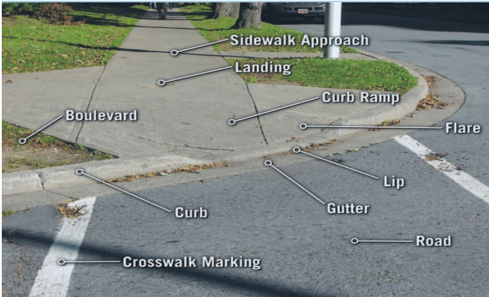
Photo Credit: Sean Bennett, Fig. 1. Representative intersection of sidewalk and road, including a diagonal curb ramp Download Scientific Figure on ResearchGate (researchgate.net)
