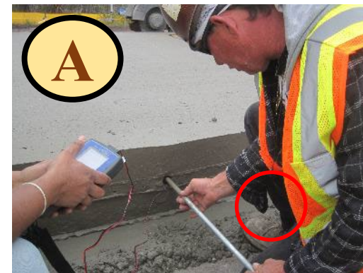
Slab edge placement
