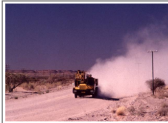
Loss of fines (as dust) on an untreated road results of applying a fines preservation treatment.
