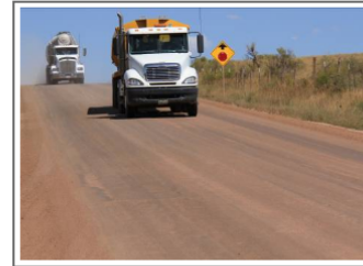
Stable fines preservation on a treated road
