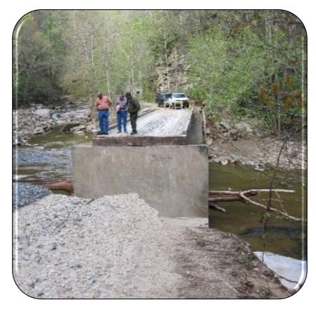
Inspection of Bridge Approach Embankment Washout during Flooding, New River George National Park, WV
