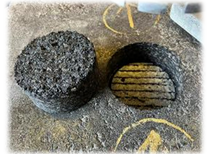
Top Layer Debonding During Coring Process
