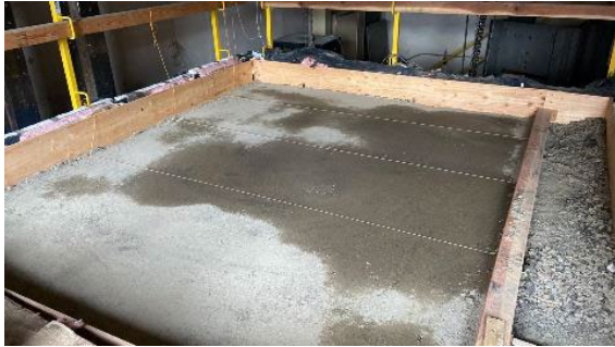
Leveling Aggregate Base Course Surface
