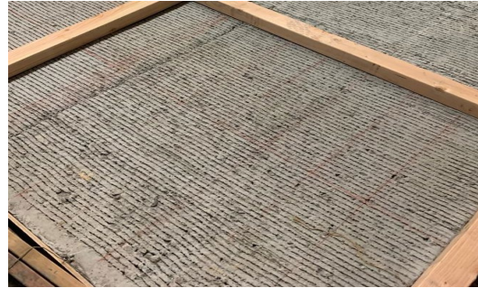
Tining the PCC Surface \approx New PCC Field Condition
