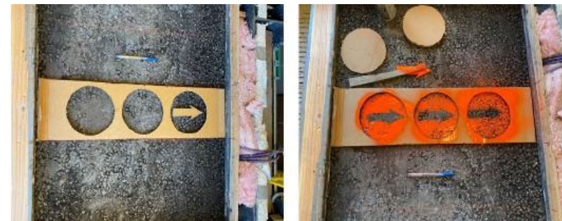
Compact New AC Layer and Mark the Tining Direction
