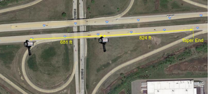
Loop, parallel entrance ramp
