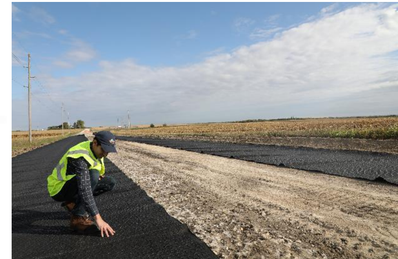
Recycled Plastic Composite Geosynthetic
