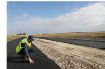
Unpaved road test section stabilized with composite geosynthetic made from 100% upcycled polypropylene in Buchanan County, Iowa, with Araz Hasheminezhad, left
