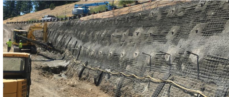
Source: Geo-Stabilization International Soil Nailing
