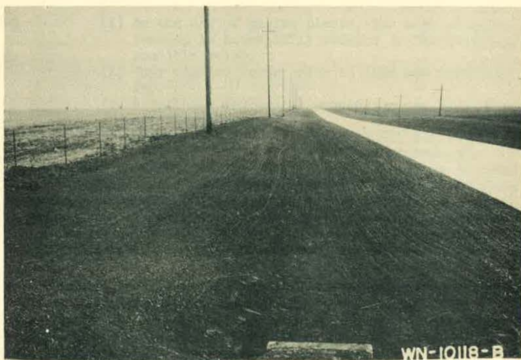
Cross section revised and area seeded to grass. Soil Conservation Service
