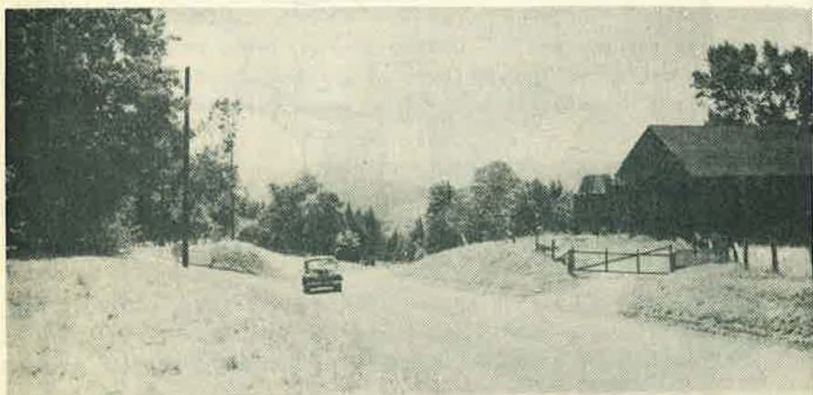
Figure 3. Typical cool, humid conditions here permit bluegrass-fescue types of sod, to become established within one season, by seeding on mulched lightly topsoiled slopes. Because of difficulty of machine mowing these steep slopes, this sod will be permitted to gradually become converted to a ground cover of native aster, goldenrod and blueberry, Sumac or sweet fern types of shrubs.
