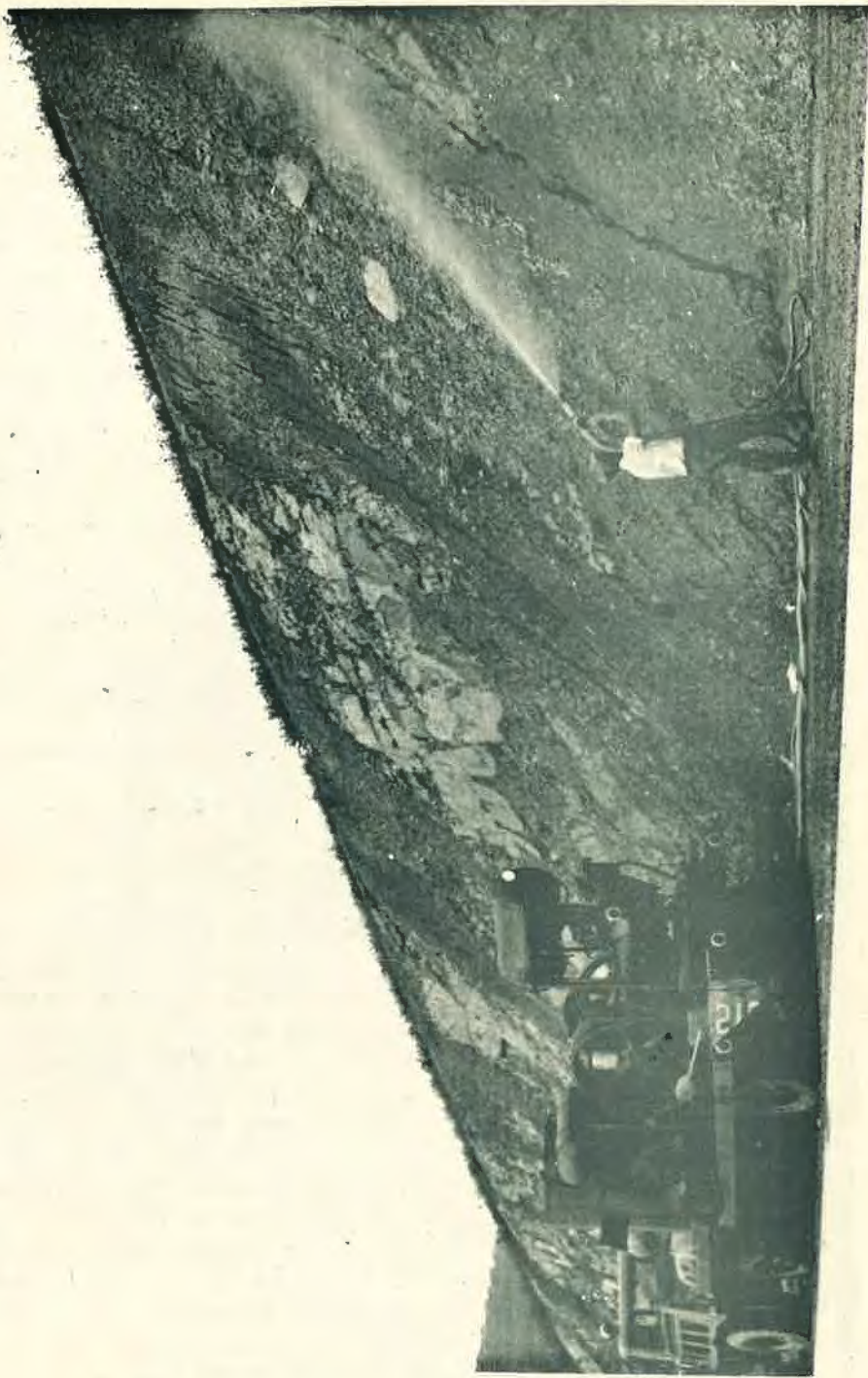
Figure 1 - Seeding Operations on the Pennsylvania Turnpike
