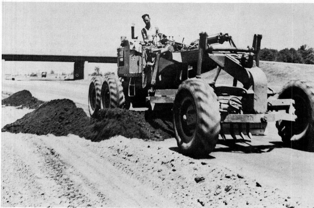
Figure 8. Bulk flyash being spread by motor grader, N. J. Turnpike project.
