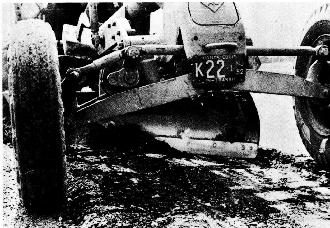
Figure 7. Preparation of shoulder for treatment. Blade is removing loose bituminous material. This operation is followed by scarifying to desired depth with the motor grader, N. J. Turnpike project.
