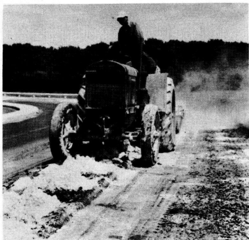
Figure 9. Mix-in-place Pulvimixer incorporates the lime and flyash into the existing shoulder. Lime was supplied in 50-lb. sacks and dropped on shoulder as shown, N. J. Turnpike project.
