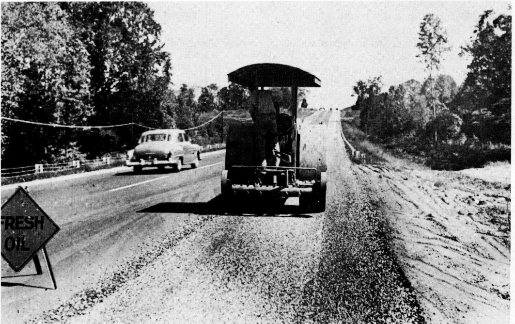
Figure 17. Application of stone chips over shoulder project at US 301, Marlboro, Md.
