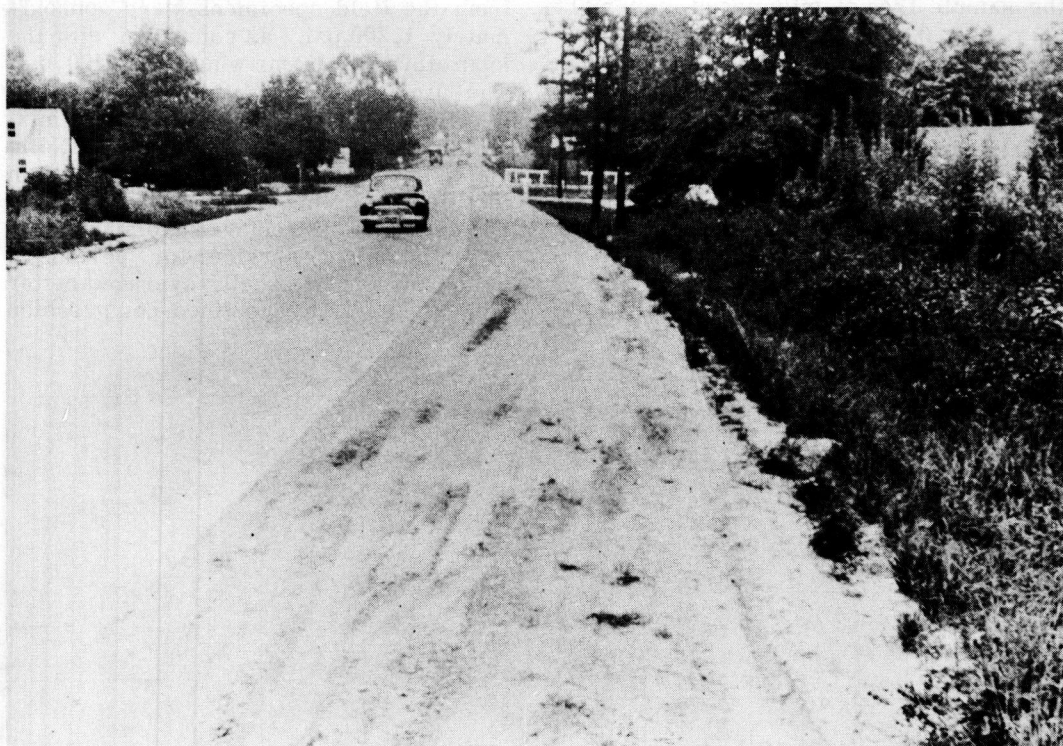
Figure 19. Condition of shoulder adjacent to stabilized section. US 1 Bypass, Laurel, Md.
