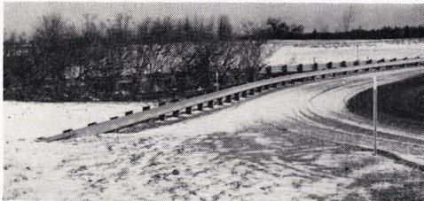
Figure 20. Proving ground standard guardrail end treatment.
