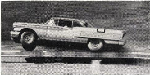
Figure 19. Impact on 37-ft sloped end.
