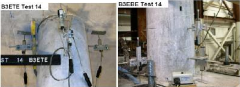
(b) Damage on the upper and lower portion of Bent-3 after T-14
