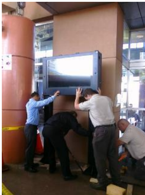
Figure 13 Passenger Information Sign Installation at LYNX Central Station
