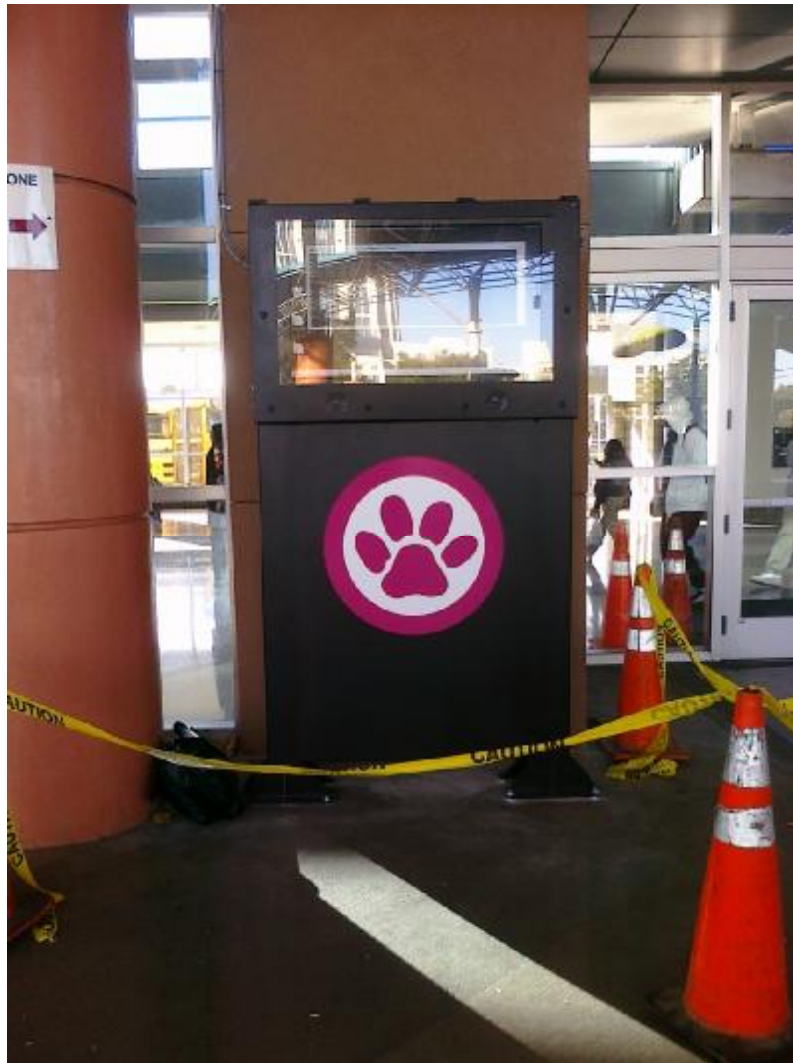
Figure 14 Newly Installed Sign Showing Glare Problem
