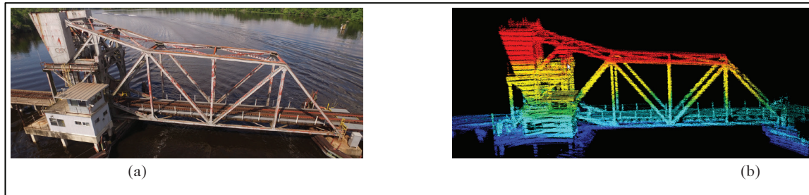
Figure 3: (a) CSX's railroad drawbridge; (b) 3D model of drawbridge from LiDAR data.
