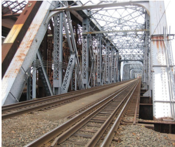
Figure 1: Span 7 of the Devon railroad bridge showing the open deck floor system and the truss structure.
