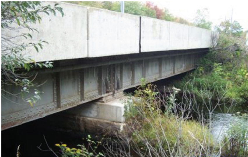
Figure 1: Amtrak Bridge 155.85 over Usquepaug River, Rhode Island.
