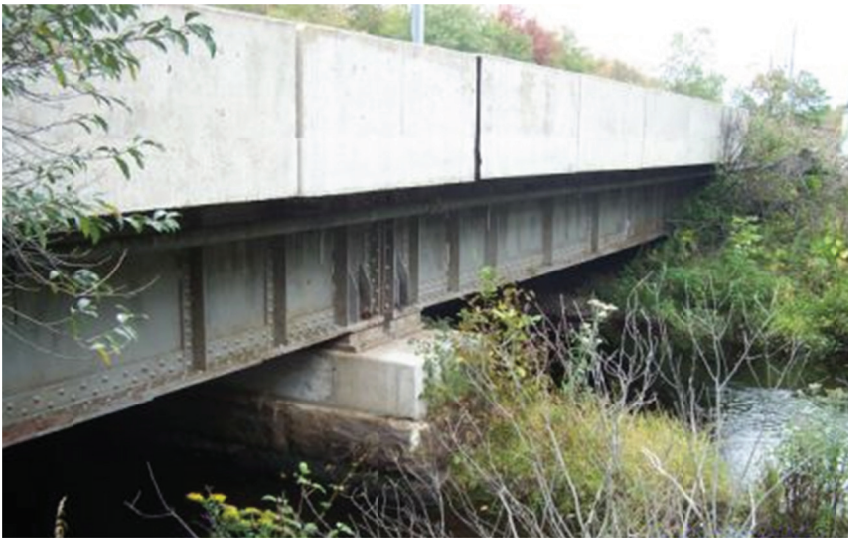
Figure 1: Amtrak Bridge 155.85 over Usquepaug River, Rhode Island.
