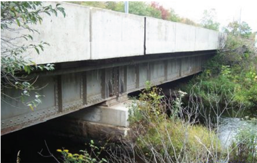
Figure 1: Amtrak Bridge 155.85 over Usquepaug River, Rhode Island.
