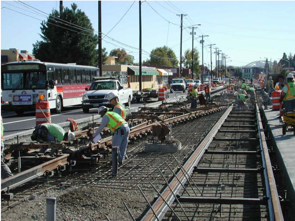
FIGURE 4 Interstate MAX light rail construction workers—track work.
