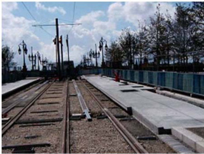
FIGURE 6 Station transition point.
