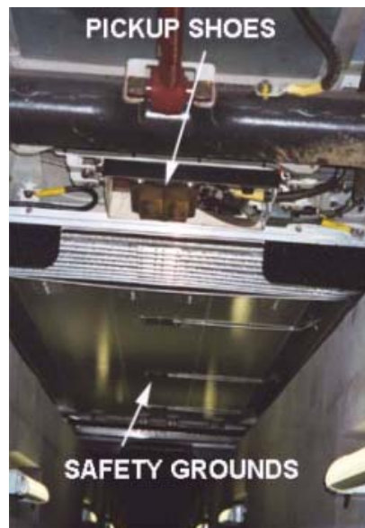
FIGURE 17 Shoe gear installation.
