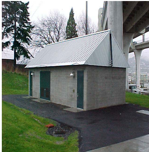
FIGURE 6 TriMet Interstate MAX LRT Graham Street Substation, 2003.
