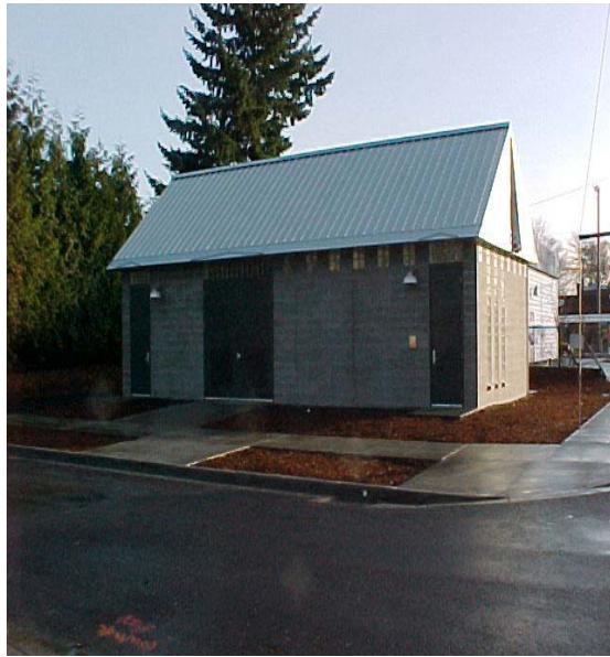
FIGURE 7 TriMet Interstate MAX LRT Killingsworth Station Substation, 2003.
