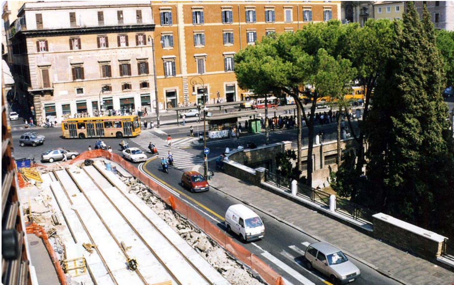
FIGURE 11 Side and central precast concrete slabs have been laid and joined to the precast concrete platform in Piazza di Torre Argentina.
