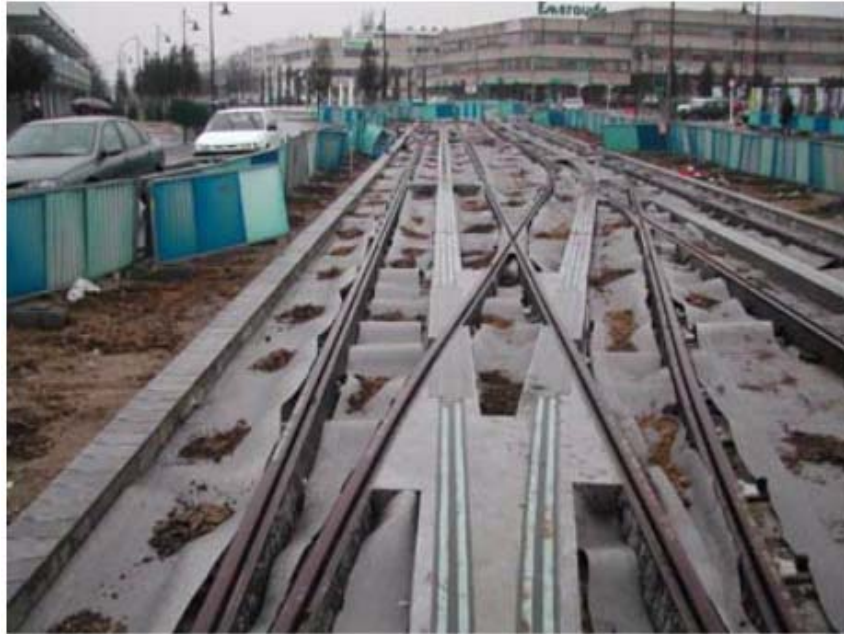
FIGURE 7 Crossing special trackwork.
