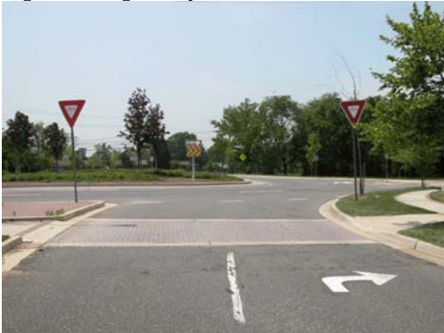
FIGURE 5 Five pavement marking turn restrictions.
