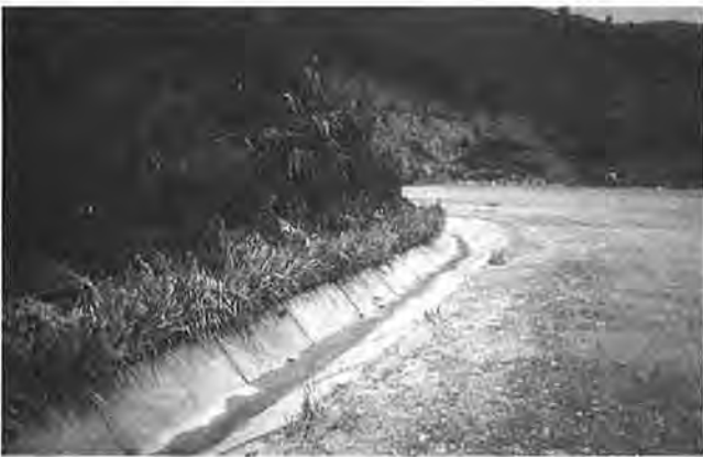
FIGURE 10 Vetiver used to protect edge of road drain from sedimentation and small rock fill in Doi Tun, Thailand. Note clean drain, which saves annual maintenance costs and ensures that drain functions when needed (photograph by R. G. Grimshaw).
