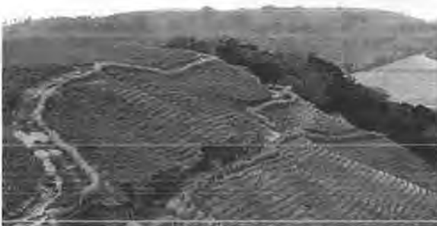
FIGURE 6 Vetiver hedge rows protecting sides of farm access roads in South Africa (photograph courtesy J. C. Greenfield).
