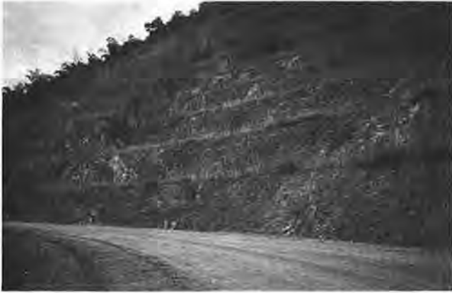
FIGURE 9 Steep, high road cut in Doi Tung Royal Development Project, Thailand, is being stabilized with vetiver hedges (1 year old). On closer inspection one sees volunteer natural species being established behind hedges where there is more moisture. Note that vetiver hedges spread out runoff, dissipate concentrated hydraulic forces, and allow runoff to move slowly and evenly down face of cut (photograph by R. G. Grimshaw).
