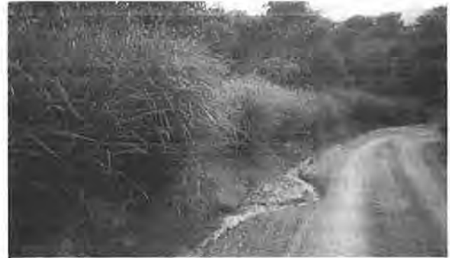
FIGURE 7 Vetiver hedges used in Guatemala for more than 20 years to protect cut slopes of coffee estate roads (photograph by R. G. Grimshaw).
