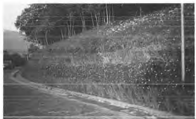
FIGURE 8 Two rows of vetiver hedges interplanted with leguminous cover effectively protect road cut in Thailand. Note sediment-free drain (photograph by R. G. Grimshaw).
