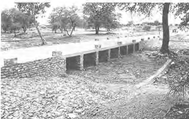
FIGURE 3 Stone masonry bridge (note guide blocks on deck and gabions and cut-off wall in foreground).
