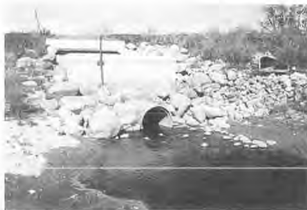
FIGURE 2 Cottonwood River box inlet structure.
