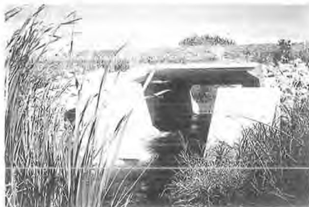
FIGURE 1 V-notch weir.
