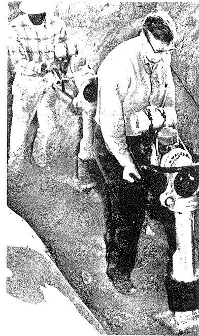
IMPACT COMPACTOR —Powered by gas engine, it jumps up and down.
