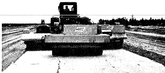
PROGRESSIVE METHOD —On thin lifts, smaller machines get good results while working at high speeds. Above, vibratory rollers are drawn by rubber-tired tractor.
