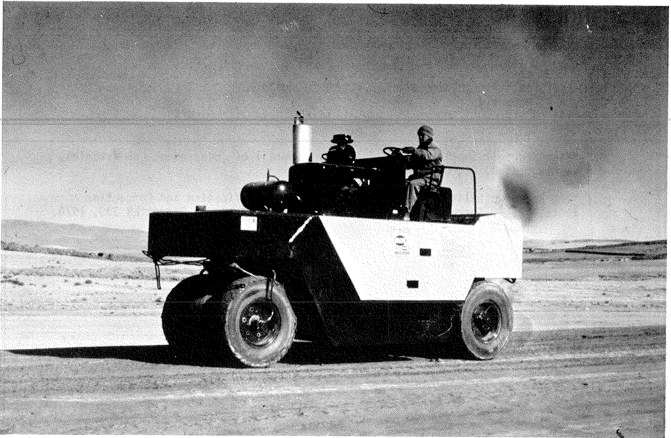
218 A self-propelled rubber-tired roller is used in construction work (Bolivia).
