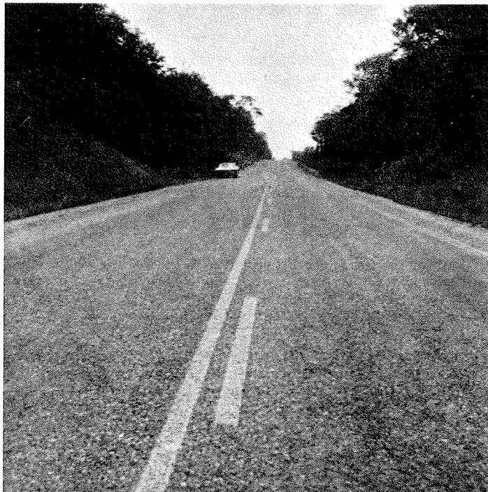
Fig. 31. Canada. Illustrating the Excellent Appearance of a Double Surface Treatment on a Consolidated Granular Base, in Its Third Year of Service, that Was Designed and Constructed in Accordance with the Principles Described in the Paper.
