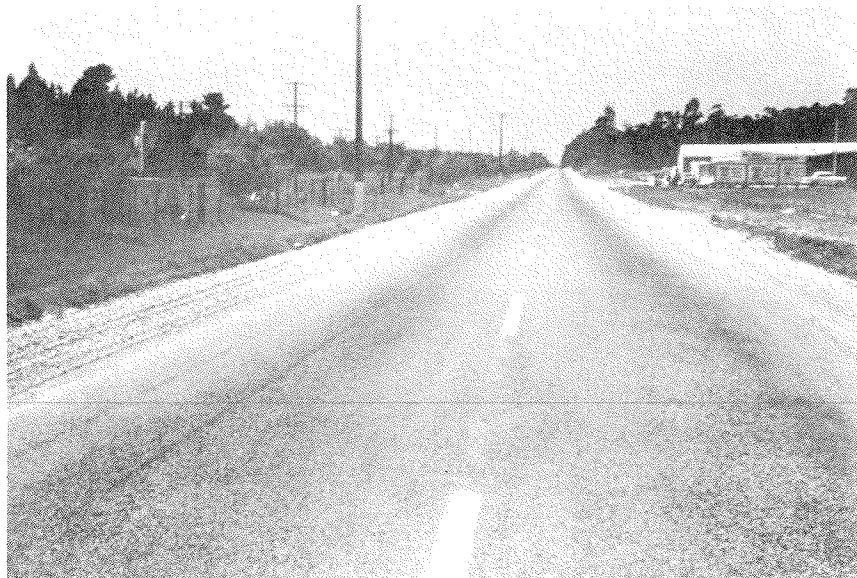
Fig. 1. New Zealand. Double Surface Treatment on Consolidated Granular Base, 15 Years Old, Carrying 3000 Vehicles per Day. Excellent Condition.
