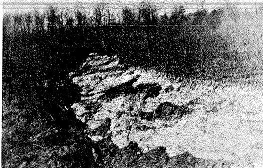
Figure 2.11. Thin layer of residual debris that slid on inclined strata of metasilstone along I-40 in Cocke County, Tennessee.
