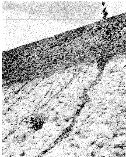
Fig. 46 Slope partly treated and partly untreated
