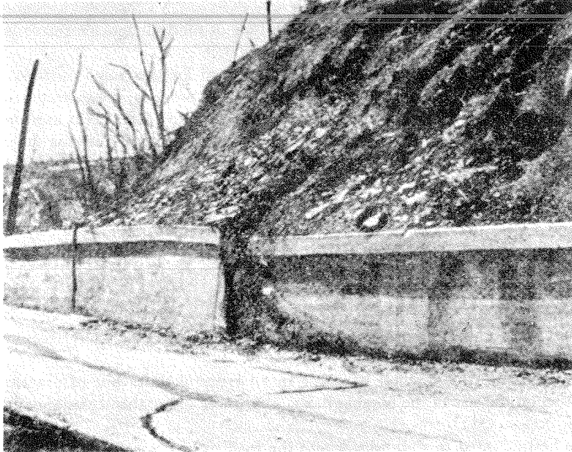
Fig. 40 Retaining wall as a protection of the road
