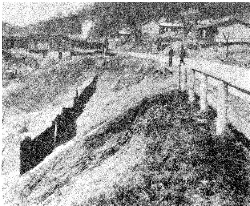
Fig. 50 Steel sheet piling to hold the embankment
