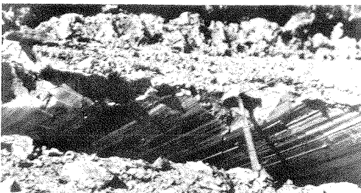
Figure 2.9. Slickensides in foot area of shallow slide in Pennington shale residuum (highly weathered clay shale) along I-40 in Roane County, Tennessee.
