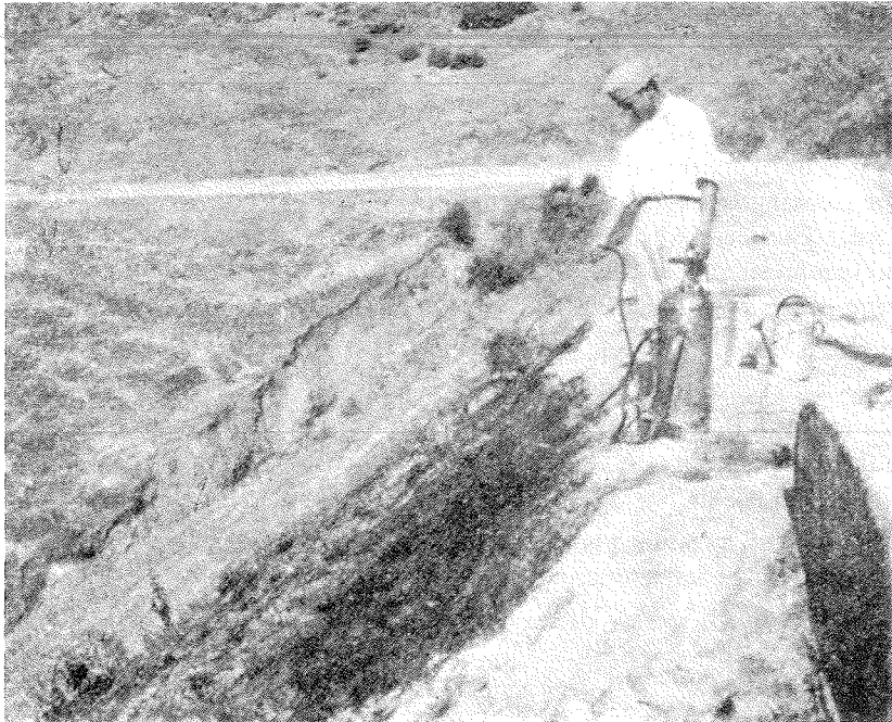
Fig. 43 Spraying of bituminous emulsion
