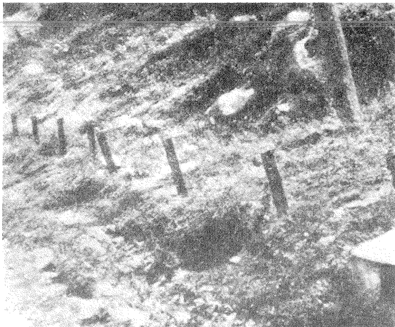
Fig. 49 Steel rails used to hold a slide
