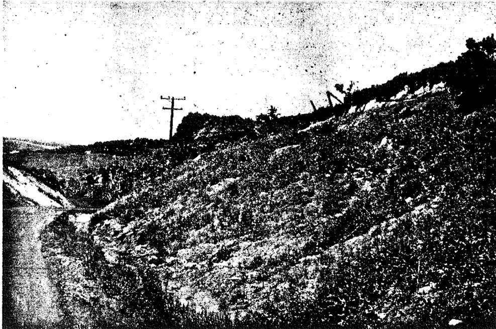
Figure 55. Ground view of a typical slide on a cut slope shown in Figure 54. (Photograph by Donald J. Belcher)
