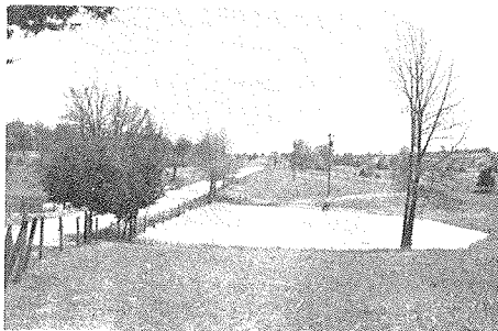
Figure 12. Topography of Limestone Area, North-Central Harrison County, Indiana (10) - Roads constructed across plugged sinkholes give poor performance because of water-logged subgrades. Flooded conditions during wet weather result in the roads being impassable for periods of several days at a time.
