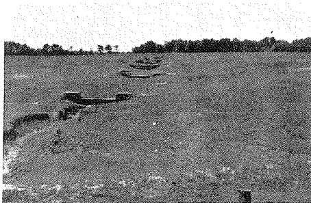
Figure 19. Erosion Control in Illinoian Glacial Drift Region, Jennings County, Indiana - At the extreme right-center, the very light tones of gray mark the silty edges of a lateral gully.
