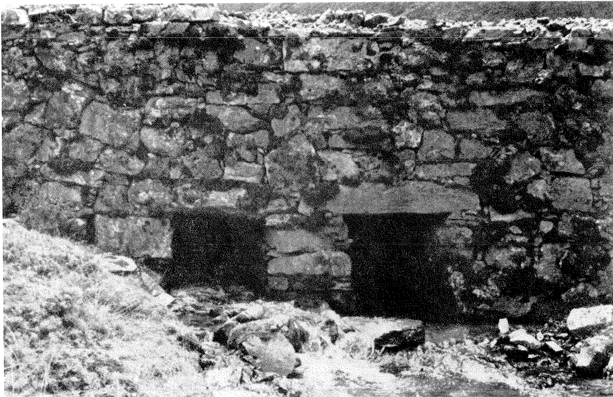
Cover photo: Dual stone box culvert in Bolivia.
