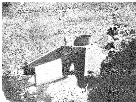
Figure 43. Concrete debris fin and metal pipe debris riser in conjunction with single corrugated metal pipe culvert.
