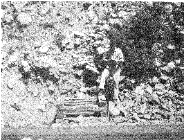
Figure 38. Timber debris crib of inexpensive local materials.
