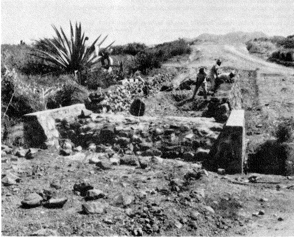
Masonry culvert is under construction in Oaxaco, Mexico.
