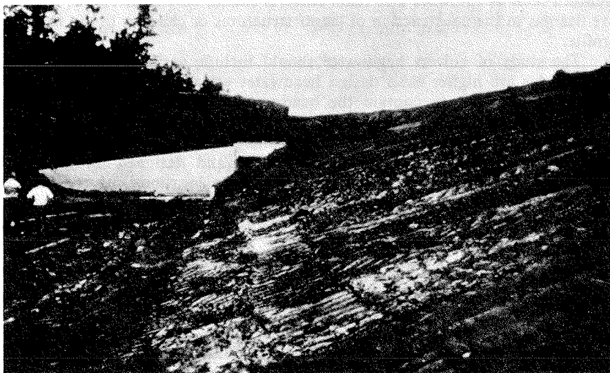
Fig. 5—Fill warped to fit culvert headwall normal to culvert.
