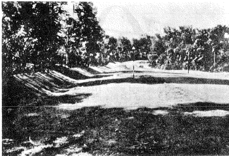
FIG. 5.6. Properly shaped and well maintained road cross-section in Kenya.
