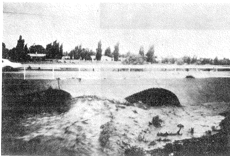
Fig. 13—Mitered inlet with slope paving.
