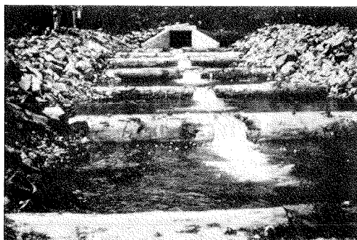
Fig. 28—Weirs downstream of culvert to facilitate fish passage.
