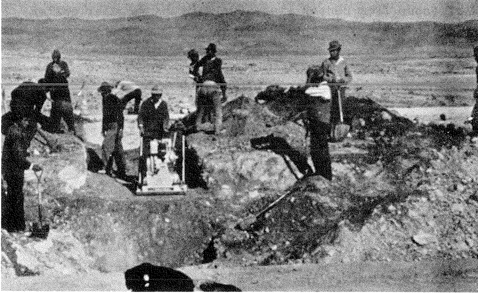
Backfill is compacted over corrugated metal pipe—Bolivia.
