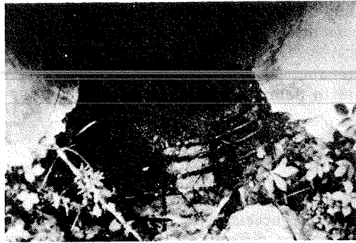
Fig. 30—Loss of culvert material from abrasion.
