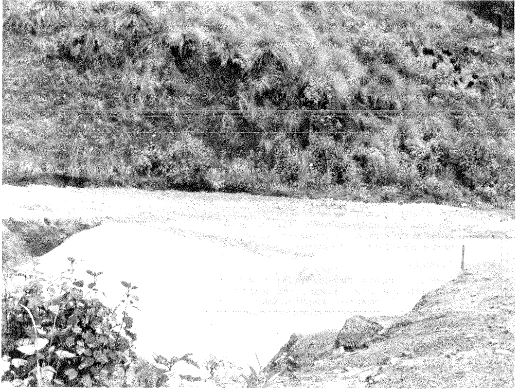
Paved dip near Oaxaca, Mexico.
