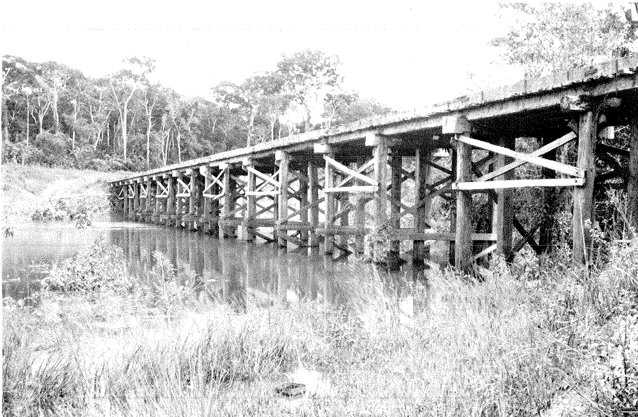
Cover photo: 104-m timber bridge, Rio Preto, Brazil.
