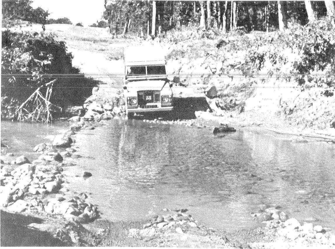
28 Temporary drift (ford), East-West Highway, Nepal. (Photo courtesy of TRRL, UK)
