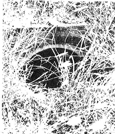
Culvert filled with Growth
