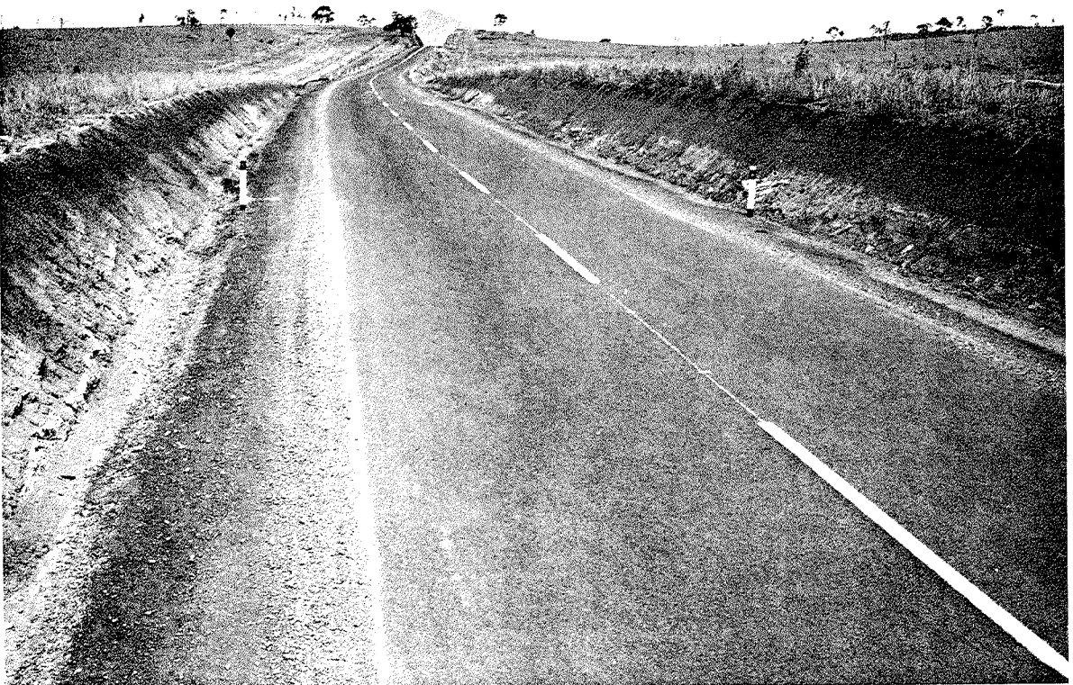
Well Maintained Table Drain
