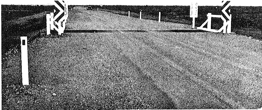
Cattle Grid (A well installed and maintained cattle grid on an open surface road)
