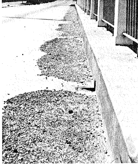
Remove Debris from Bridge Deck
