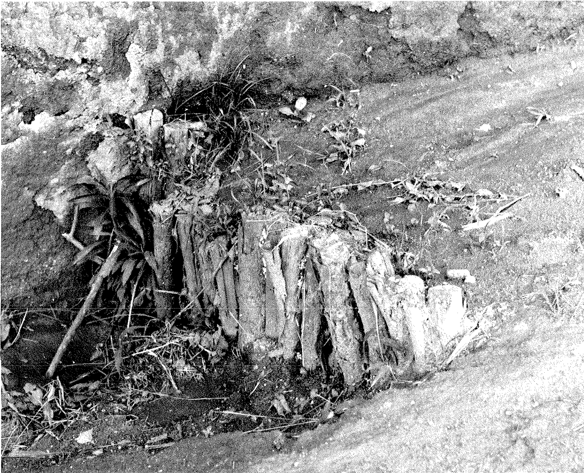
Ditch check constructed of driven wooden stakes, Kenya. (Photo courtesy of TRRL, U.K.)
