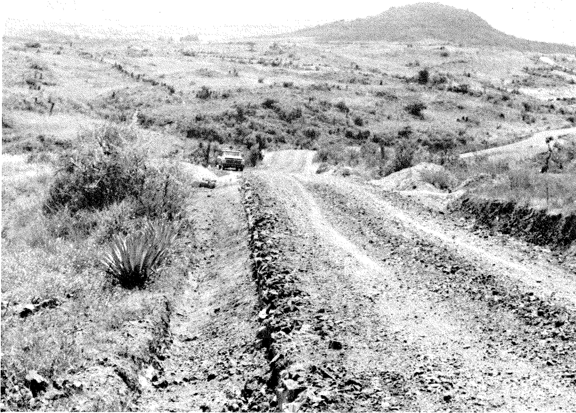
Typical roadside drainage channel constructed with labor-intensive methods, Oaxaca, Mexico.
