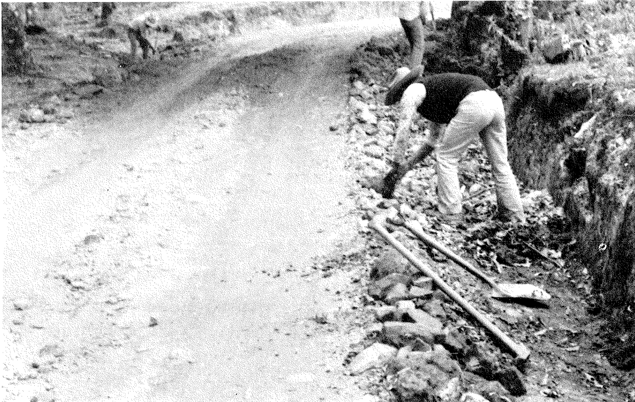
Cover photo: Labor-intensive ditch maintenance, Oaxaca, Mexico.
