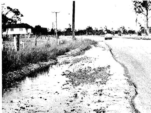
Debris on Shoulder
