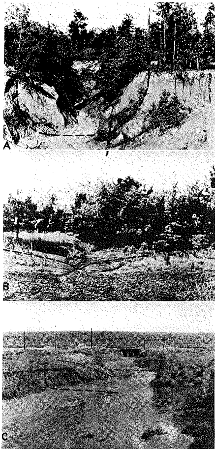
Figure 27. An illustration A, of gullies in sandy soils and, B, in claypan soils. The U-shaped gullies are short and begin abruptly—photo taken at head of gully. V-shaped and flat angle-shaped gullies in the more plastic soils extend well into the upland on a more uniform gradient. C: A typical gully found in arid regions where “flash floods” attack dry soil banks and often create U-shaped gullies in clay soils.
