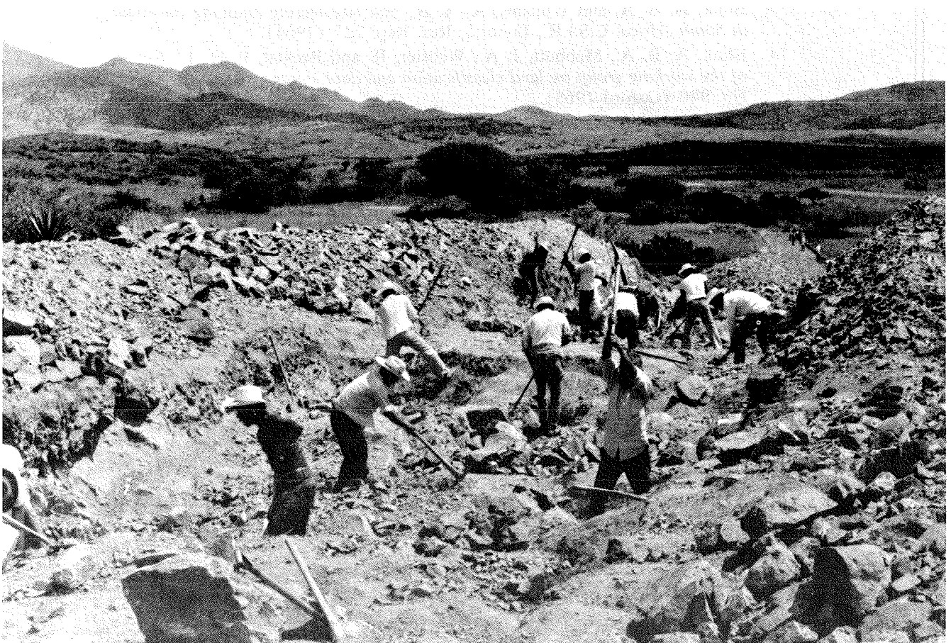
Rock excavation in a cut section, Mexico.
