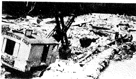
Figure 11. View Showing Tightly Cemented Boulder Formation Predicted from Seismic Tests at Pemigewasset River Crossing Near Lincoln, New Hampshire
