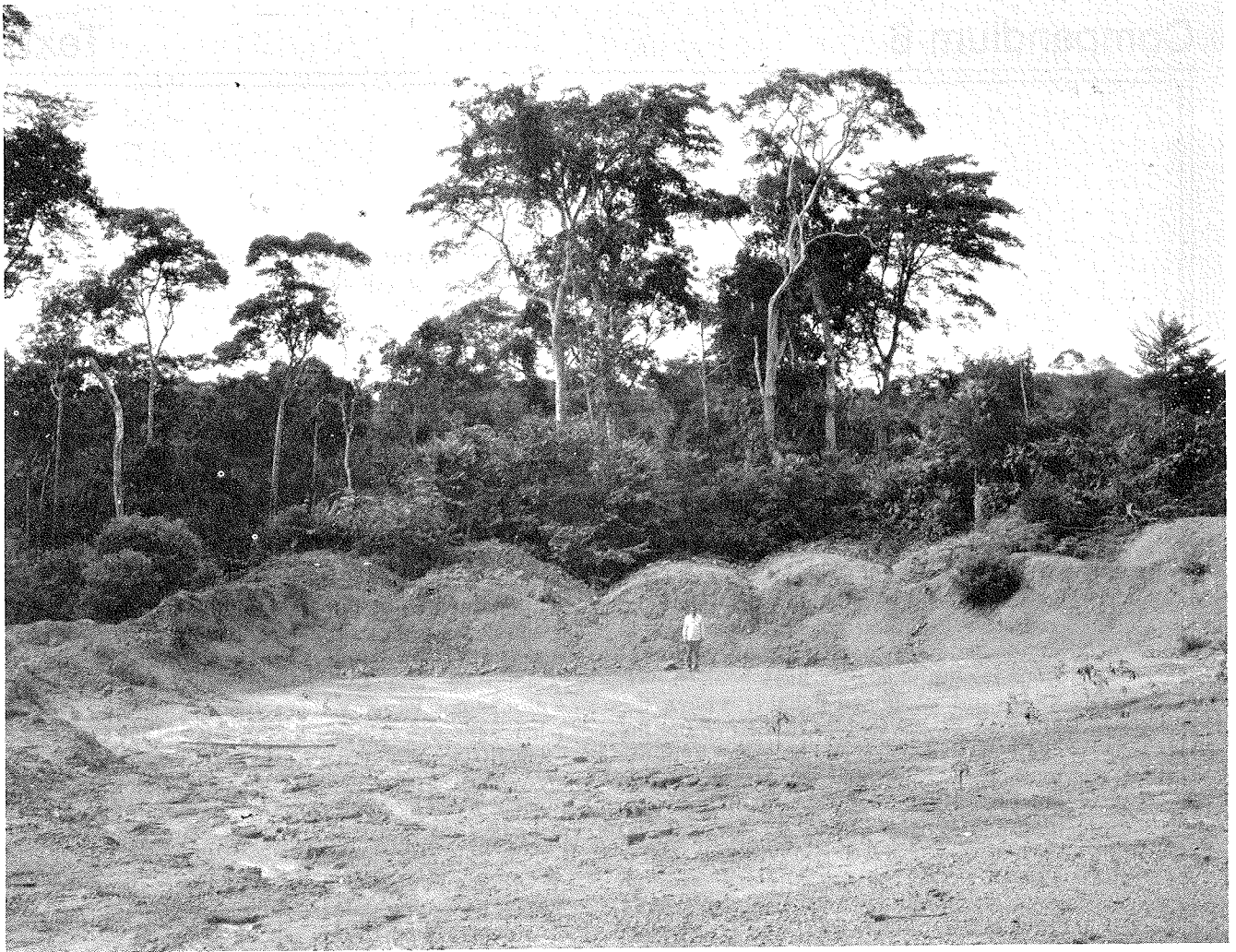
Typical borrow pit (0.6 km from roadway) with gravel used as road-surfacing material, Brazil.
