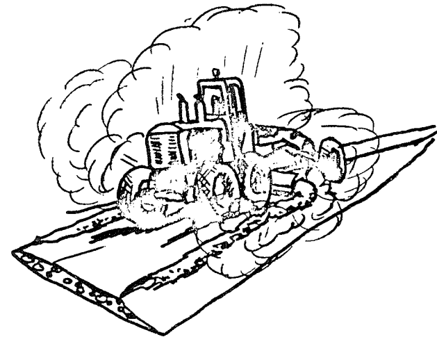
Fines Blowing Away As Dust
