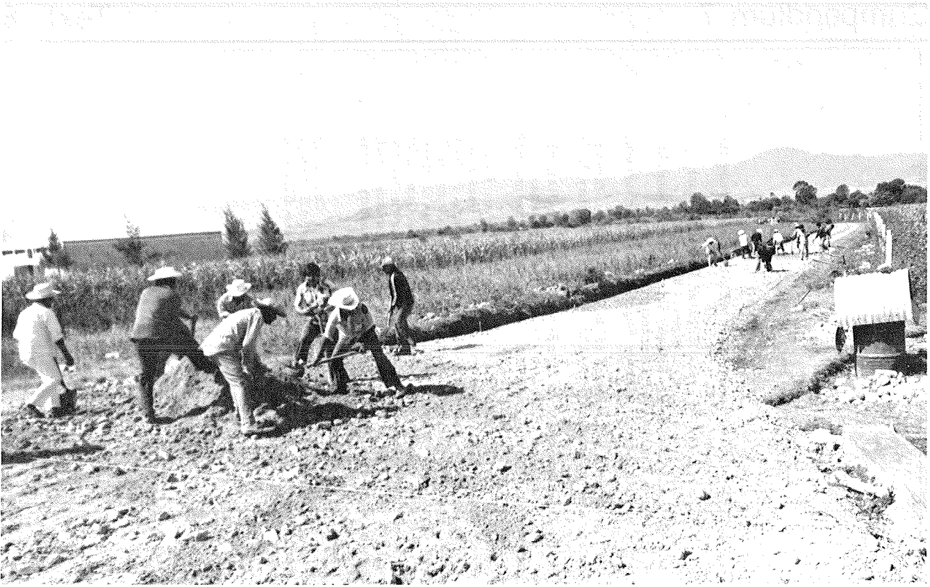
Labor-intensive construction of gravel surface in Oaxaca, Mexico.
