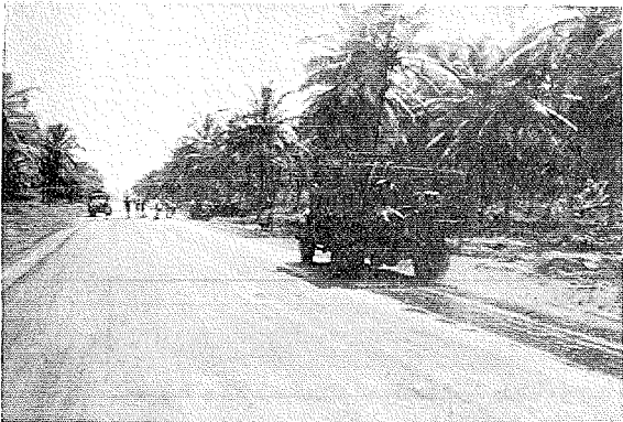
Plate 5—Curing of Soil-Cement road, with water
