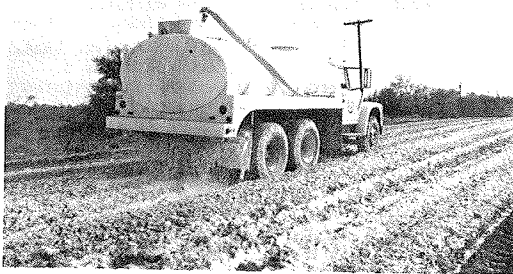
(a) Stabilization of stone base (Ref 16).
