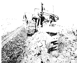
Figure 27a. Deep stabilization of access road—Dallas-Fort Worth Airport. After lime spreading the plow cuts to a depth of 61 cm (24 inches).
