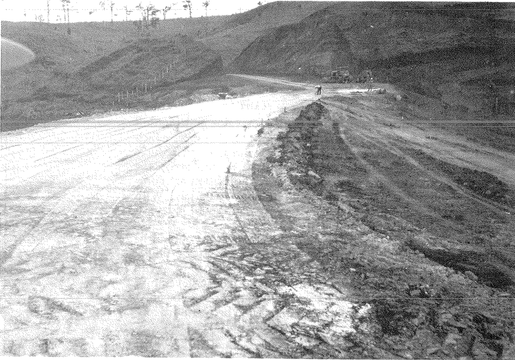
Grader blade is used to mix lime-stabilized laterite soil (Honduras).
