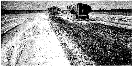
Figure 37. Watering of lime-treated clay on airport project—Kansas City, Missouri (Ref 9).
