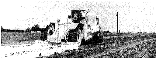
(b) Recirculation pump on top of 2.3 m 3 (6000 gal) wagon agitates slurry.
