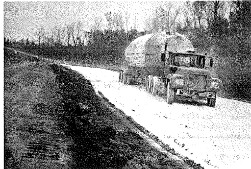
Figure 30. Application of lime by a bulk pneumatic truck for levee repair project.
