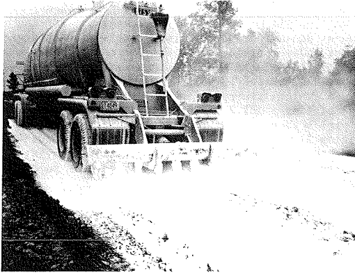
Figure 31. Distribution of lime from bar spreader-Wisconsin.
