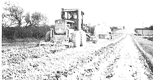
Figure 36. Grader-scarifier cutting slurry into stone base.
