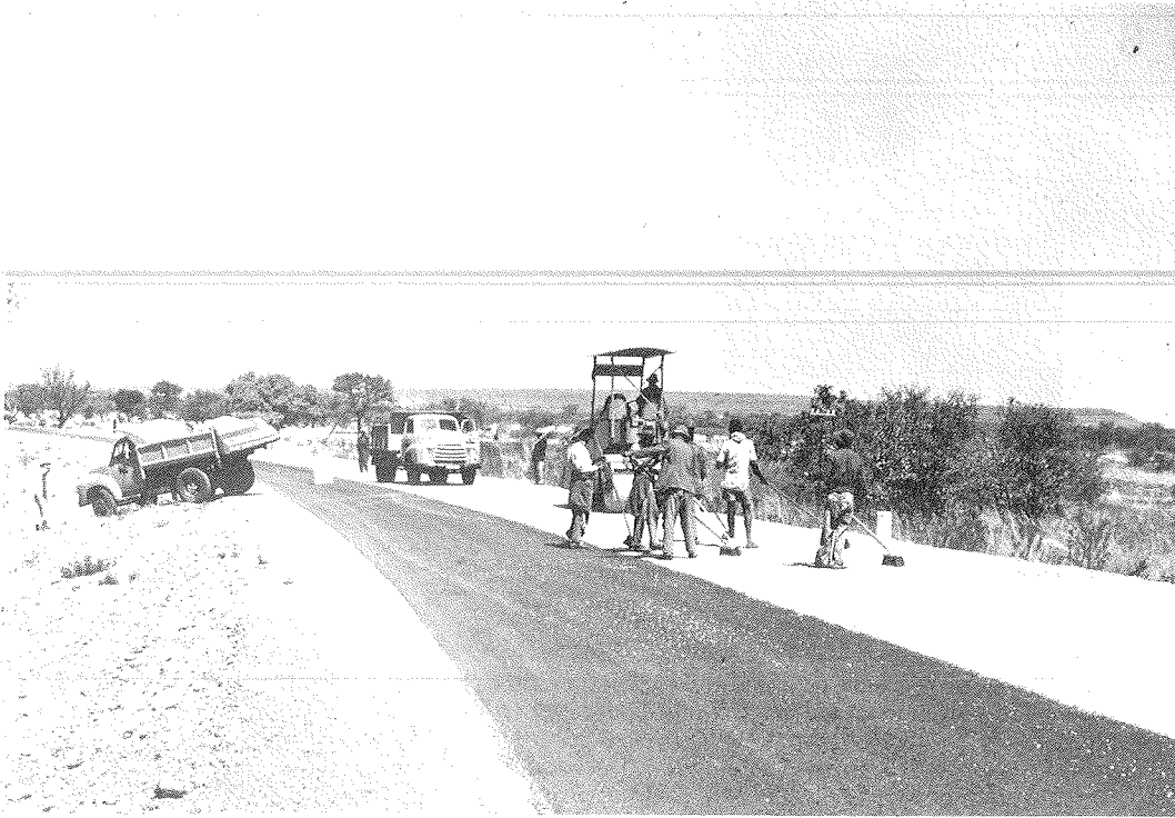
Surface treatment is applied to a lime-stabilized lateritic gravel (Central Africa).
