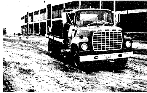
Figure 5a. Partially completed stabilized subgrade resists rutting during rain—Dallas-Fort Worth Airport.
