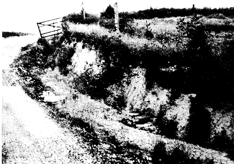
Fig. 1. A flatter cut slope would improve sight distance and establishment of vegetal cover.
