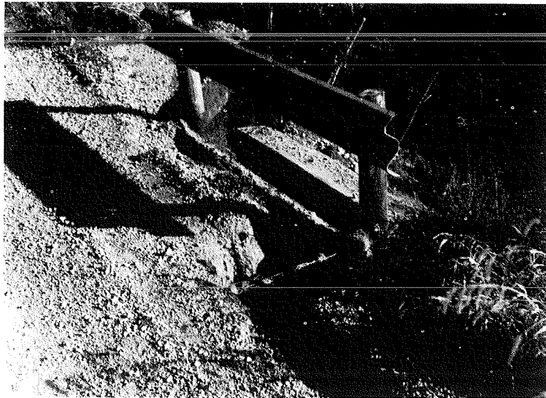
Fig. 13. Water has washed out both the original headwall here and the timber replacement. The correction of this problem is diverting the water down the side slope before it reaches the structure.
