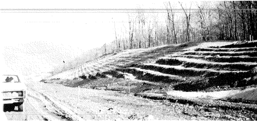
Serrated slopes aid in establishing vegetation.
