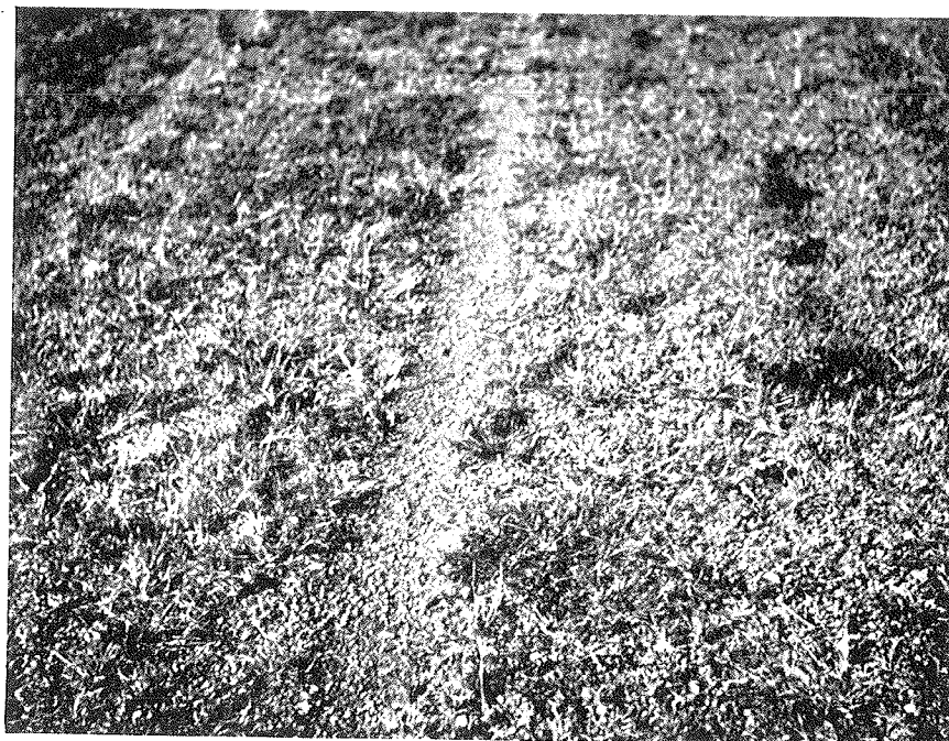
(B) The grass-bound laterite surfacing of the runway at Fort Jameson Airfield, Northern Rhodesia, showing a particularly severe skid-mark
