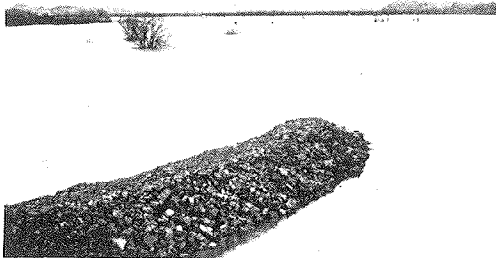
Figure 14. Rockfill spur dike near Susquehanna River bridge in Nanticoke, Penn., during 1964 flood.
