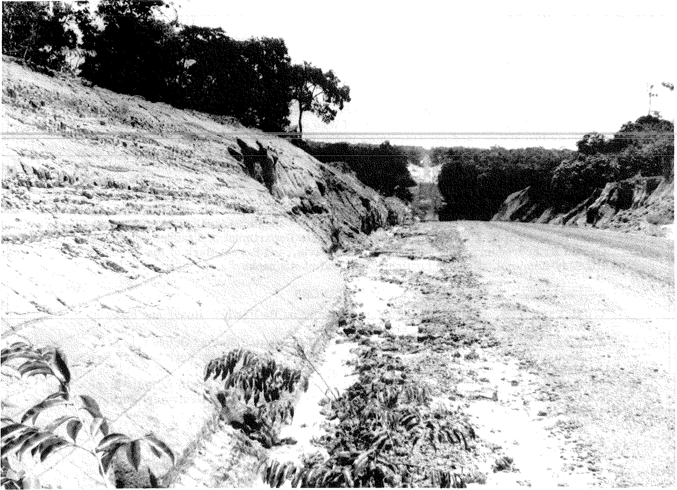
Start of erosion in side ditch where flow of water exceeds scouring velocity (Brazil).
