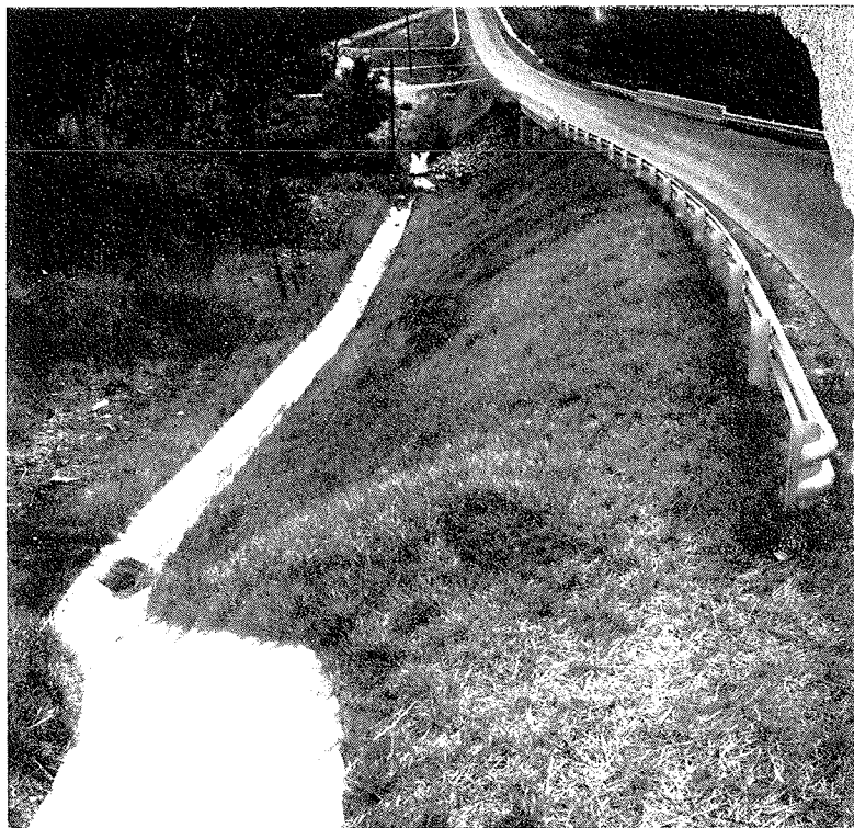
Fig. 19. An excellent example of a continuous ditch is shown here. Note culverts (top center) under each driveway, paved lining on steep sections, and the outlet to the stream.
