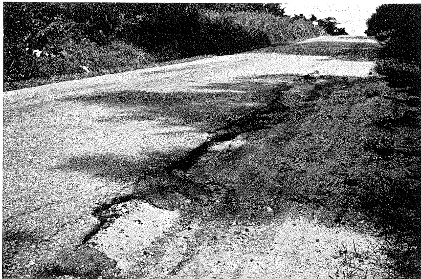
(B) 20 yards along the same road where grass is absent and fretting has occurred
