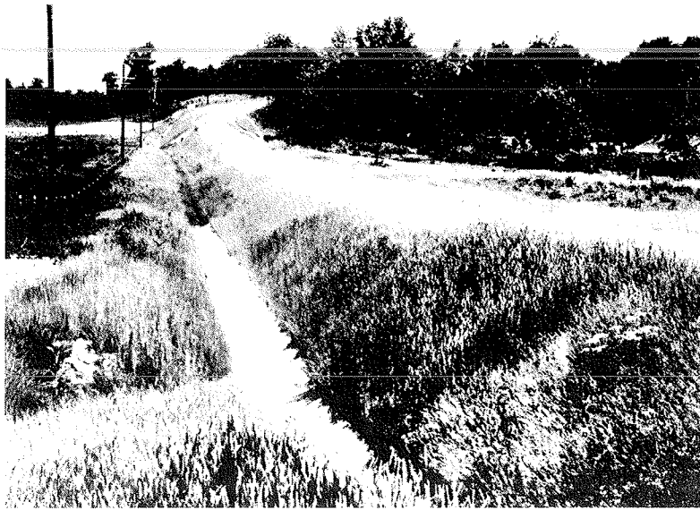
Fig. 7. Application of the principles of slope protection is well illustrated on this county road. Note the flat slopes with well rounded edges, and the turf cover over the entire slope.
