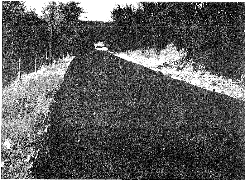
Fig. 5. A well protected slope where native woody growth has been allowed to take over.
