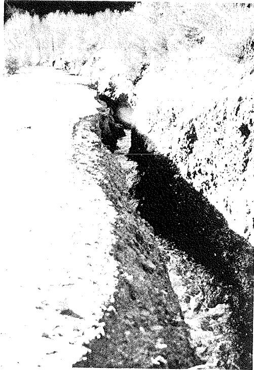
Figure 4. Deeply scoured ditch caused by failure of ditch relief culverts.
