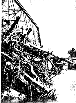
Figure 1. Debris deposited on bridge by floodwaters.
