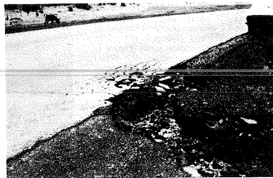
Erosion of shoulder by rain runoff from the road, with damage to pavement by headward erosion. Zone III/IV. Trucial Coast
