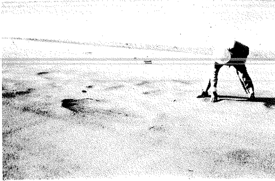
Above: Salt blisters. Jet efflux layer to a runway, Sabkha, Zone IV, Arabian Gulf
