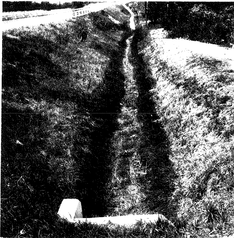
Fig. 16. A ditch and slope both protected with a healthy turf. The slopes were seeded and mulched. The thick, darker growth in the ditch illustrates the advantage of sod in providing immediate protection and more rapid development.
