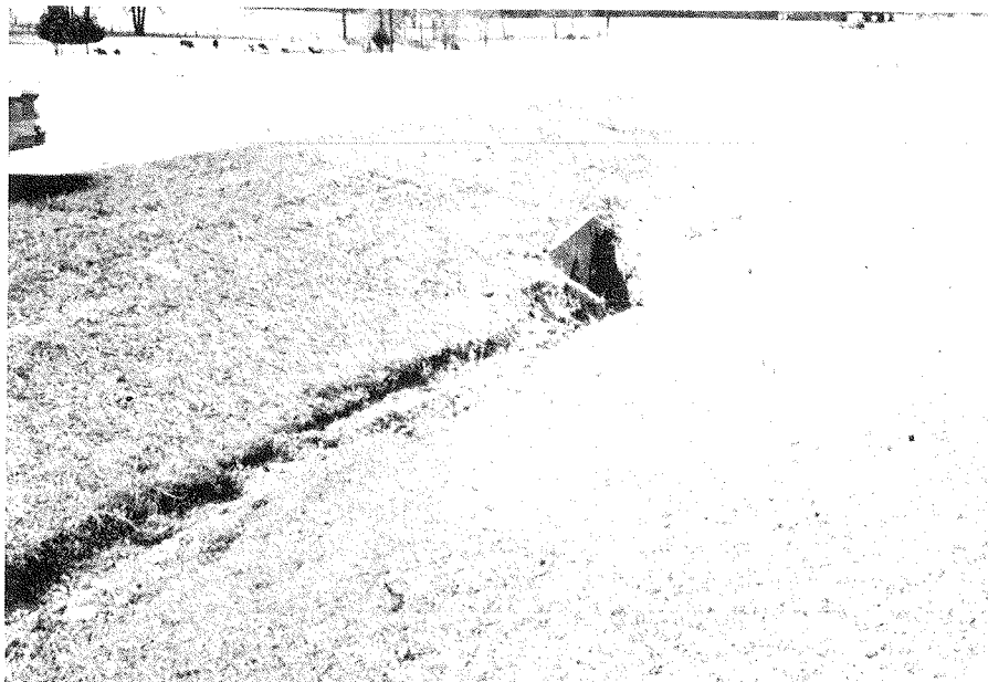
Connecting culverts in median minimizes erosion and improves safety. Median drainage can be dropped into culverts through traffic safe inlets.
