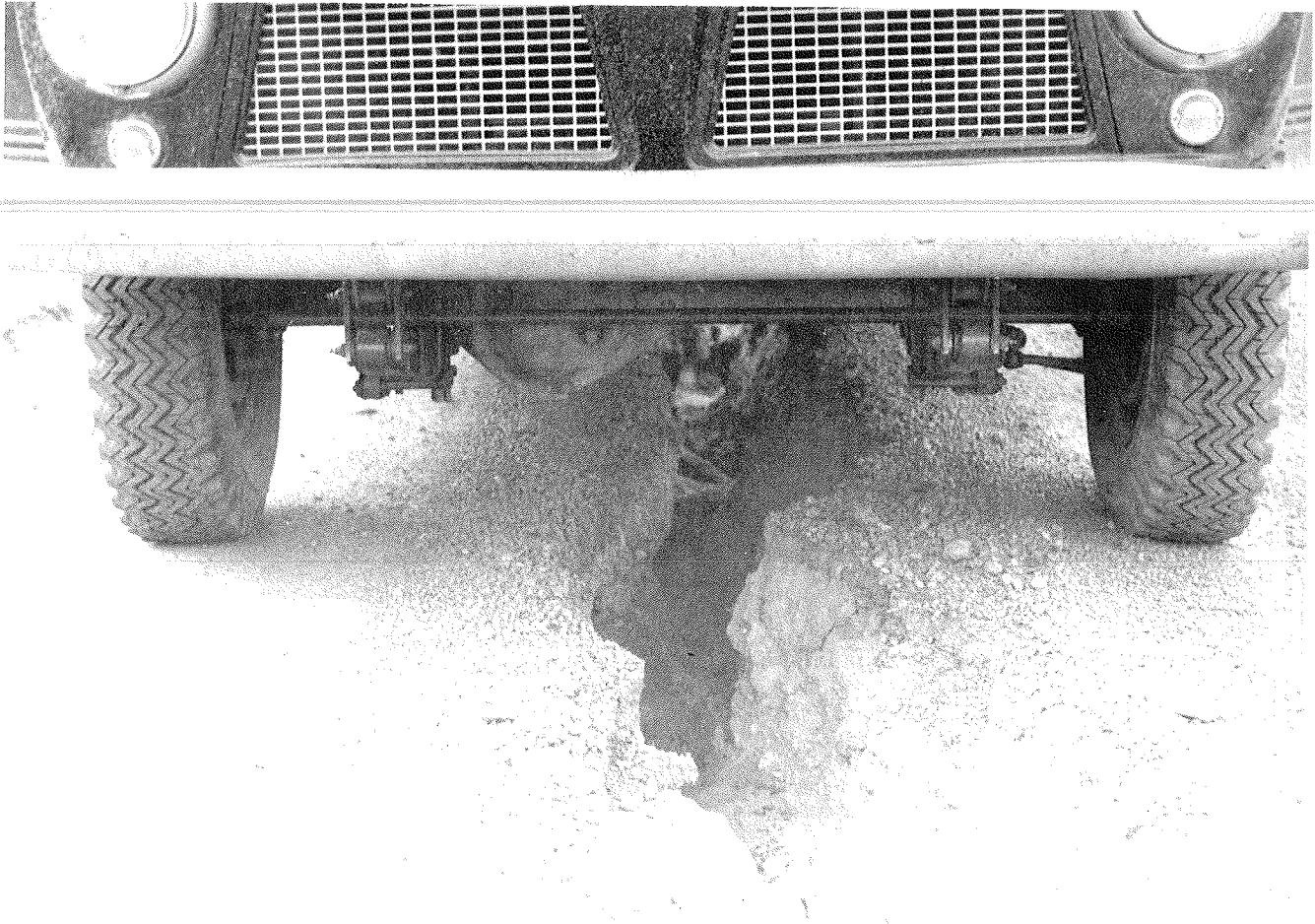
Erosion on downgrade that resulted from water running in wheel rut (Brazil).
