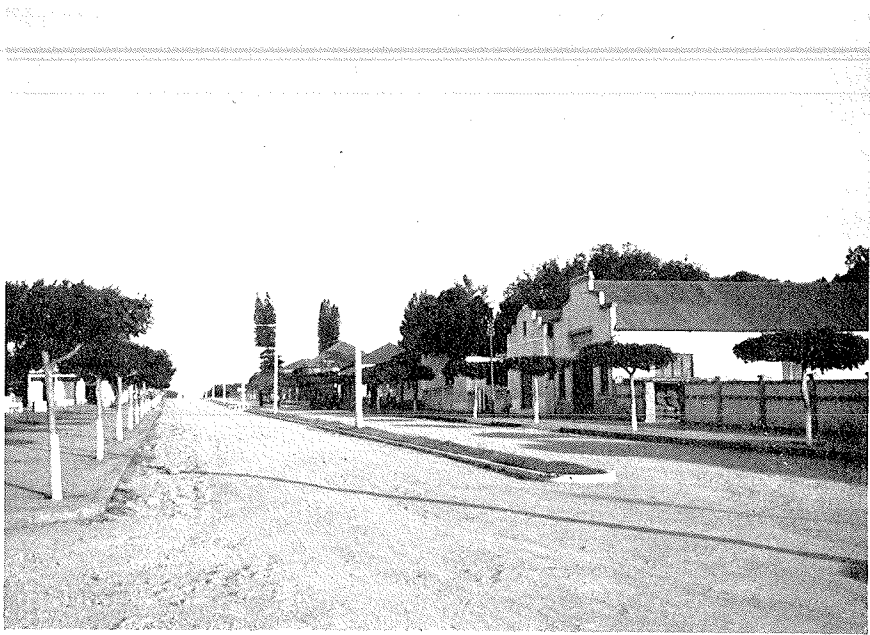
(A) White paint on tree trunks to indicate the road edge at night, in Chibuto, Portuguese East Africa
