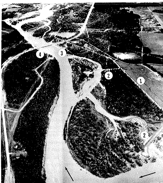
Figure 5.2 Aerial oblique photograph showing various types of training works on a braided gravel river: 1, dike; 2, spurs; 3, guide bank; 4, protected embankment end slope. (Constructed 1962)
