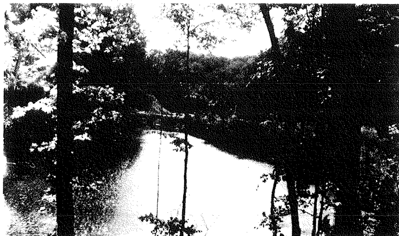
Fig. 44. This pond is created by using the highway embankment as a dam. Note the culvert outlet safely below road level at the far side of the pond.
