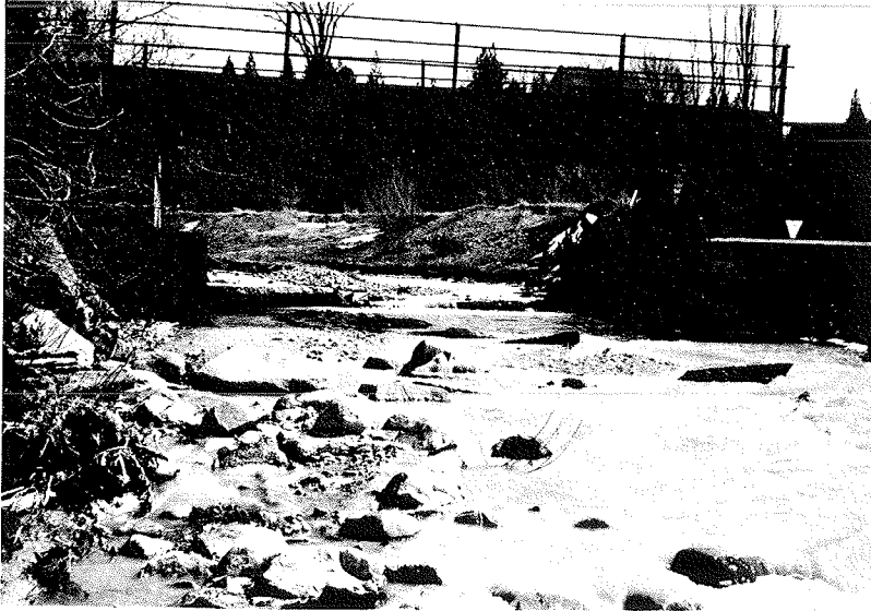
Figure 4.5 Bridge foundations repeatedly undermined as a result of progressive channel profile degradation.
