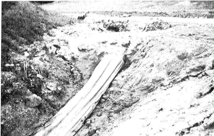
A temporary on-grade sediment basin with collapsible outfall pipe.
