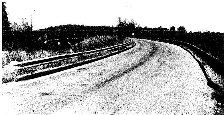
Fig. 14. Asphalt curbs contain water in this roadway, carrying it away from the structure and steep slopes.
