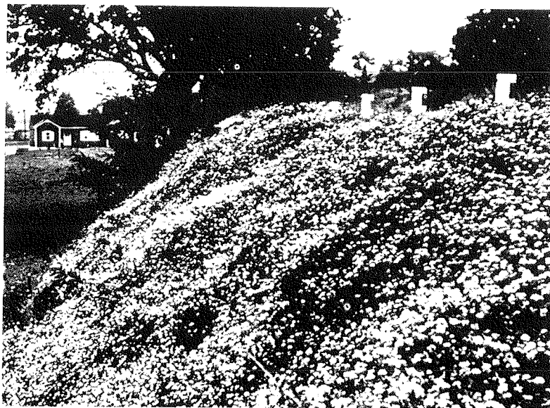
Fig. 4. The excellent protection provided by Crown Vetch is illustrated on this steep embankment slope. (Courtesy W. H. Daniels)
