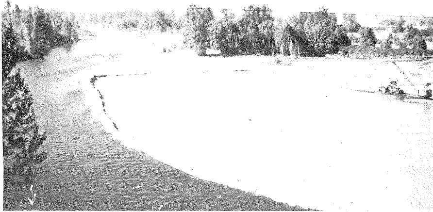
Saving fish and fingerlings is important. A dike separates "blue-water" river (at left) from borrow pit during gravel removal operation. Borrow pits in a stream should be avoided.
