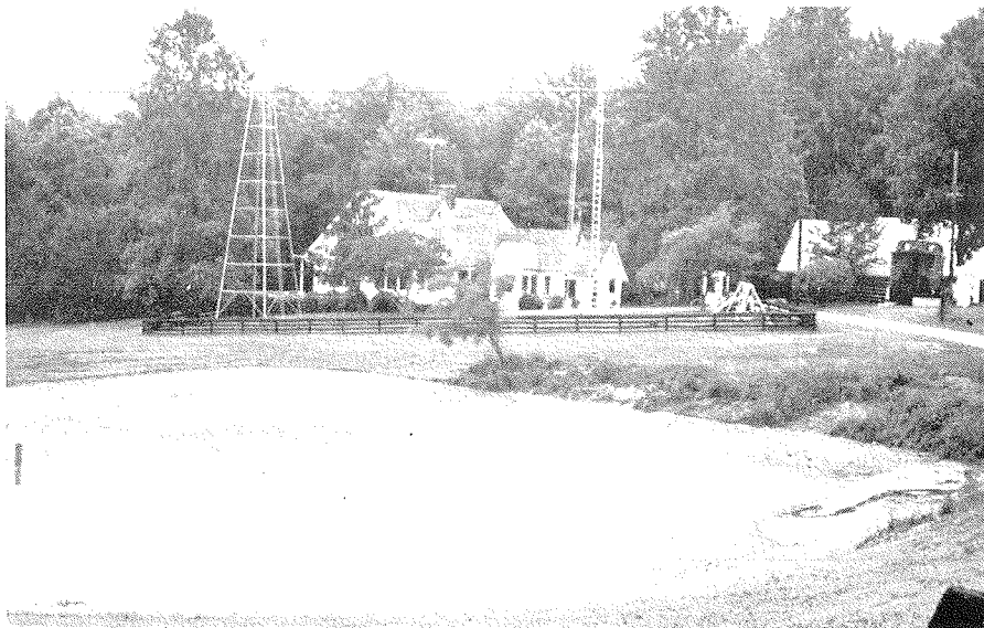
Sedimentation basin built with cooperation of landowner to catch sediment from highway project. Note riser type outlet pipe in pond.
