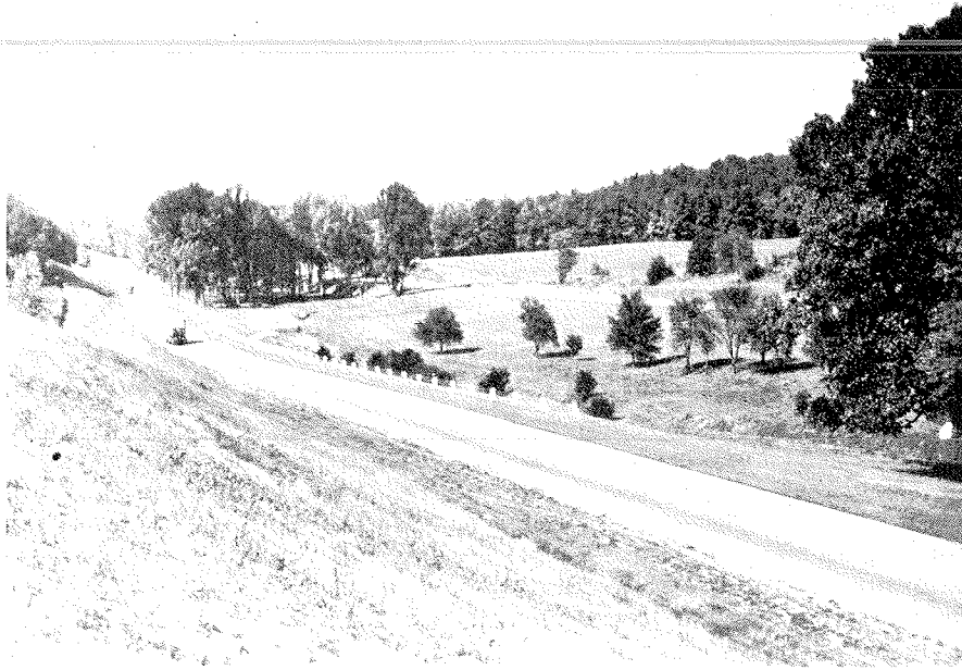
Independent roadways fitted to the landscape minimize erosion and sediment problems.
