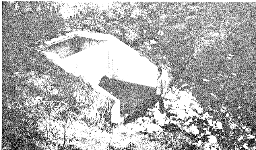
Impact type energy dissipator at culvert outlet. Some kind of protection should be provided at most culvert outlets to prevent failure.
