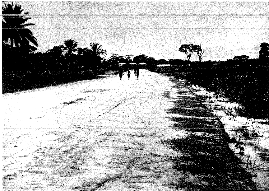
(A) Grass establishing itself on the haunches of the sand-clay road between Ughelli and Kwale in the Eastern Region of Nigeria
