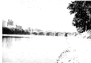
Figure 3. Arch bridges, such as the Market Street bridge in Wilkes Barre, Penn., were most damage-resistant.
