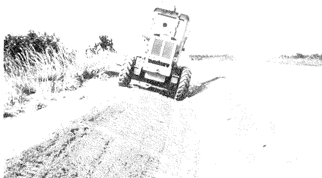
Figure 47. Machine Shaping of Ditches With Motor Grader (Ghana).
