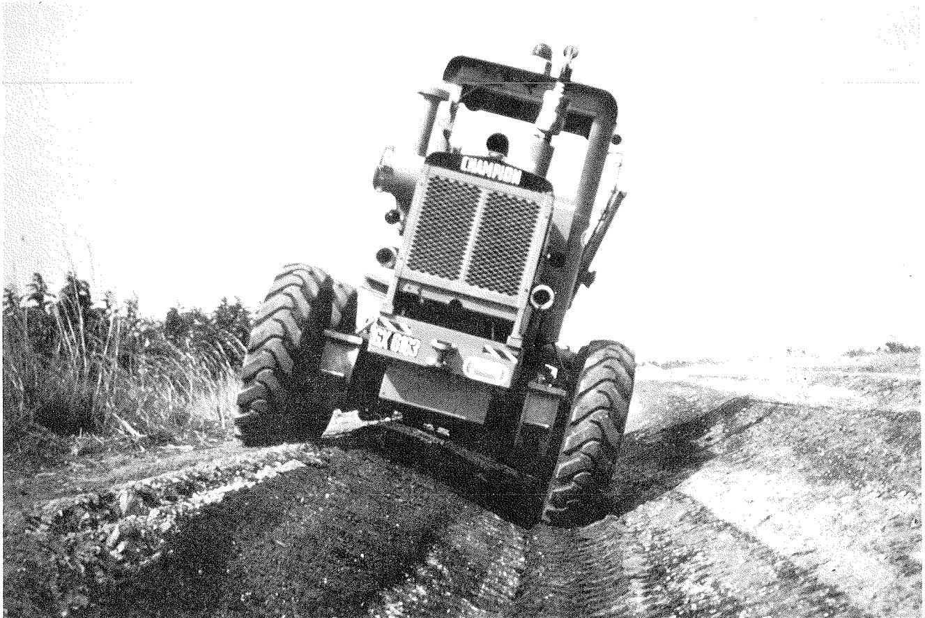
Cover photo: Ditch maintenance (Ghana).
