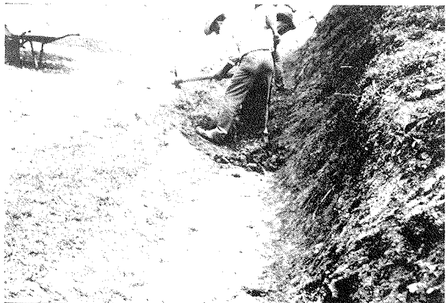
Figure 43. Typical Labor-Intensive Ditch-Cleaning Operation (Ghana).
