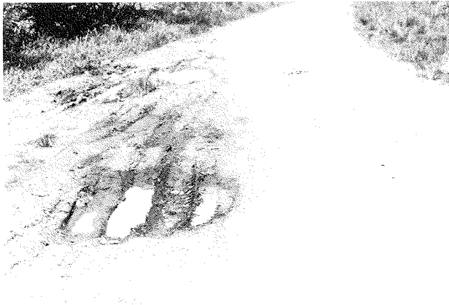
Figure 26. Unpaved Surface Deterioration.
