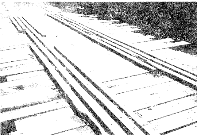
Figure 57. Deteriorated Timber Bridge Deck (Sierra Leone).
