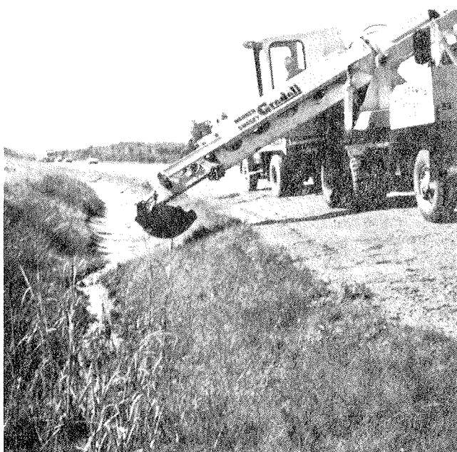
Figure 49. Cleaning Ditches by Gradall.
