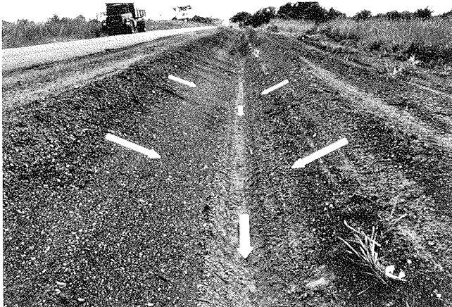
Figure 46. Example of Good Slopes and Alignment (Ghana).
