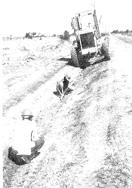
Figure 48. Checking Flow Line for Low Spots (Dominican Republic).
