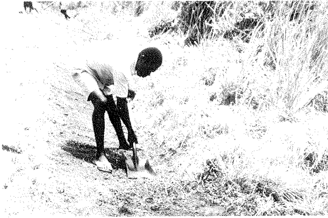
Figure 44. Typical Labor-Intensive Ditch-Cleaning Operation (Ghana).
