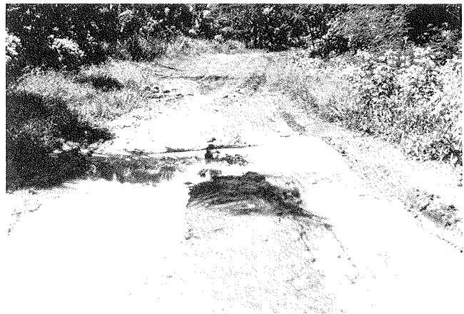
Figure 25. Unpaved Surface Deterioration.
