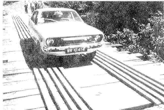
Figure 59. Completed Bridge Deck Repair (Sierra Leone).
