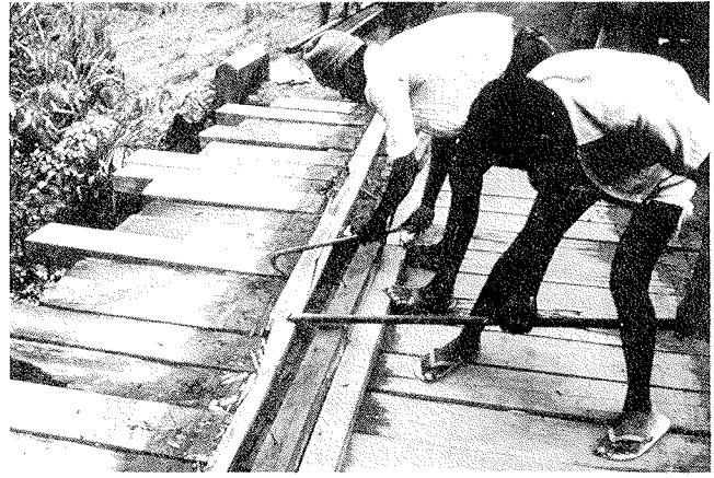
Figure 58. Deck Repairs Underway (Sierra Leone).
