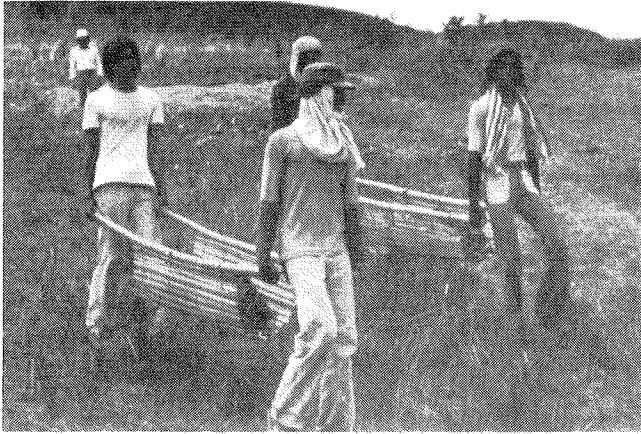
Carrying excavated materials on 2-man stretchers (Philippines)
