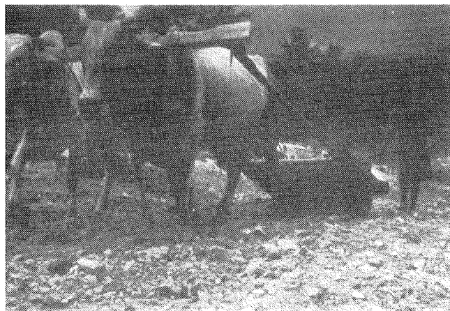
Bullock-drawn smooth-wheel roller: concrete shell at ends of oil drum to support axle, ballasted with water and weights on draw-bar with counterbalance behind roller.
