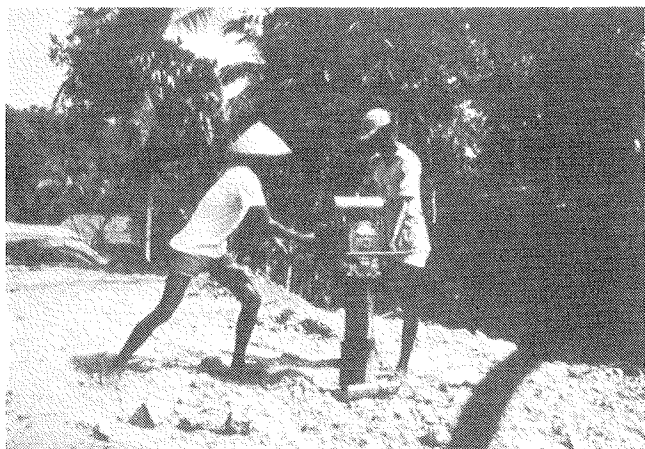
Hand-held mechanical rammer: vibratory plate at foot of column supporting power unit and steering handles.
