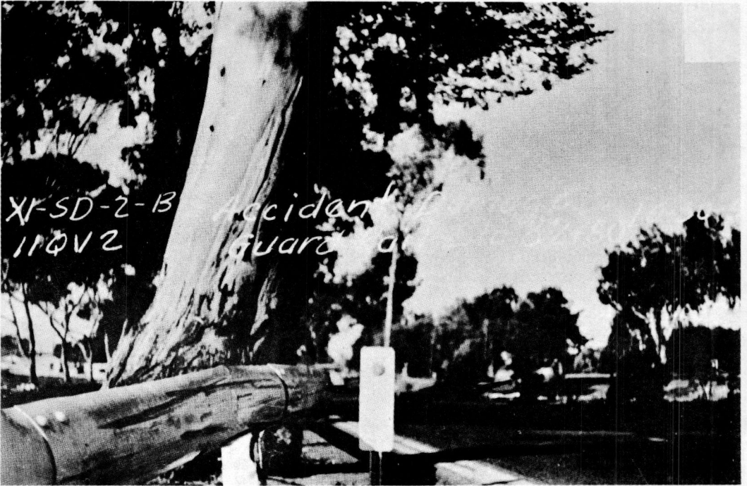
Figure 10. Steel guard rail on US 101 in California.
