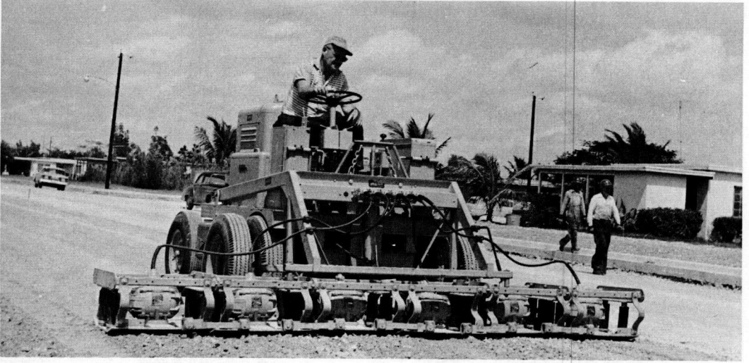
Figure 122. Multiple-unit vibrating base-plate-type compactor compacting granular base course materials.
