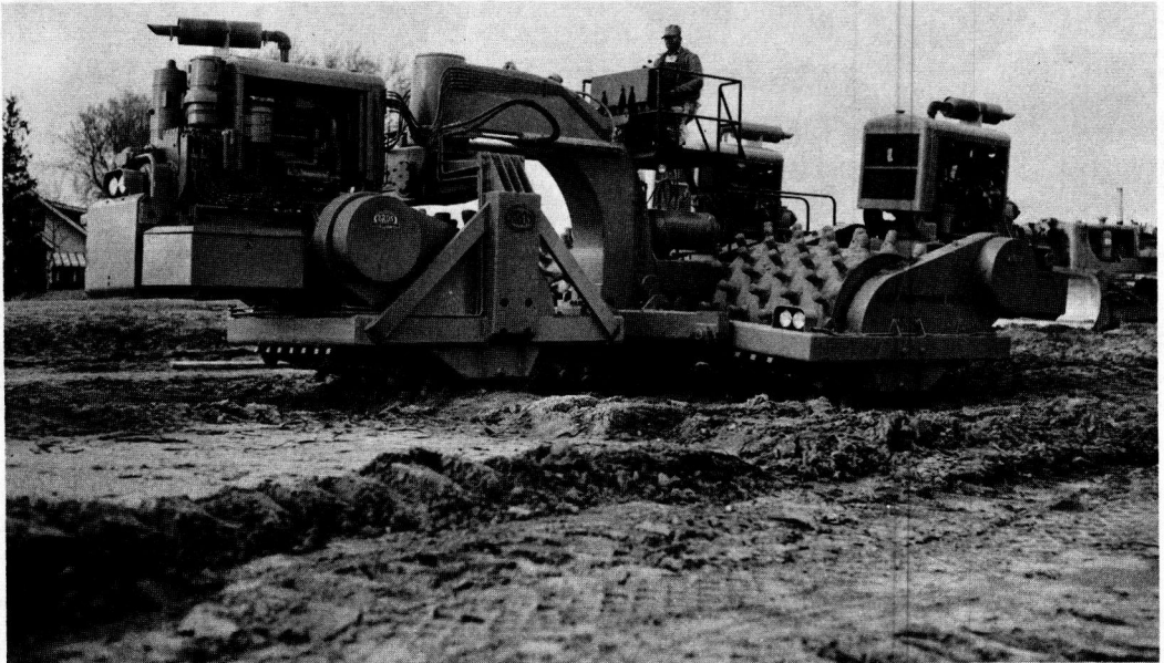
Figure 115. 40.5-ton triple-drum self-propelled sheepfoot roller.
