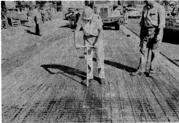
Figure 6. Using crimping tool to eliminate bulges in wire fabric.
