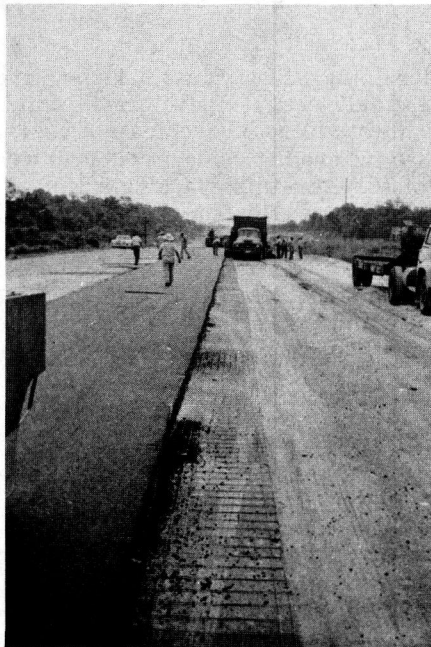
Figure 6. Same strip of fabric (Fig. 5) after surface course has been placed over one-half of it. Practically all bulges have been removed by crimping; evidence of cracking in the fresh surface course seen near exposed fabric in foreground. Note end of strip protruding through the surface course in center of photograph.
