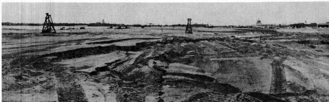
Figure 2. Fill settlement and slide planes at north side runway Stations 45-47.
