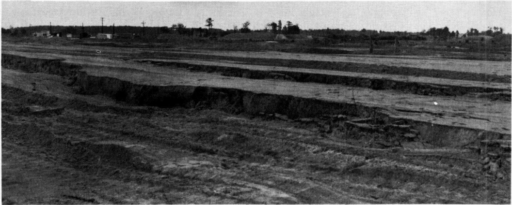
Figure 1. Fill settlement and slide planes at north side runway Stations 45-47.
