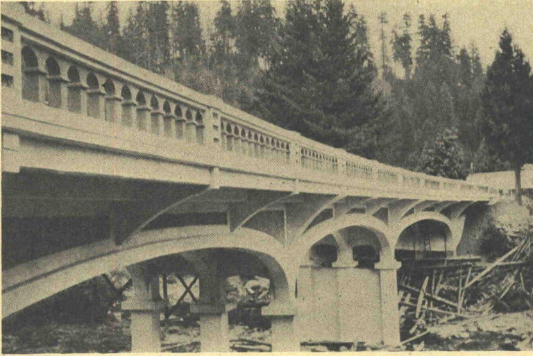
Figure 21. A Photograph of the Bridge Shown in Figure 20
